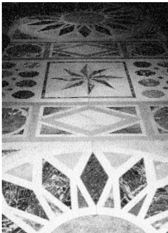
Figure 14.12 Chatsworth, Derbyshire. North corridor, 1841. Sir Jeffrey Wyattville. Marble floor by Leonardi, a Roman craftsman, working on the Forum (Photograph, Jane Fawcett)
