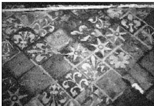
Figure 12.4 Completed mortar repairs and pointing conservation (Photograph, Cliveden Conservation Workshop Ltd)
