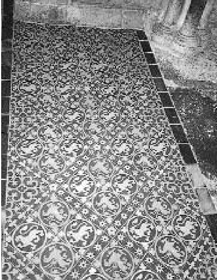
Plate 4 Salisbury Cathedral Chapter House. Encaustic tiles by Godwin, laid c.1856 during restoration by Henry Clutton and William Burges, replicating thirteenth-century tiles, recorded by Henry Shaw in 1858. Note similarities with thirteenth-century muniment room tiles – see page 6 (Photograph, Jane Fawcett)
