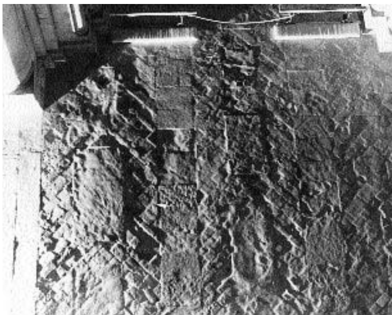
Figure 9.2 The central crossing floor illuminated by CEI, rendering the surface profile more clearly visible and showing the extent of damage and wear (Photograph, Dr C.J. Brooke)
