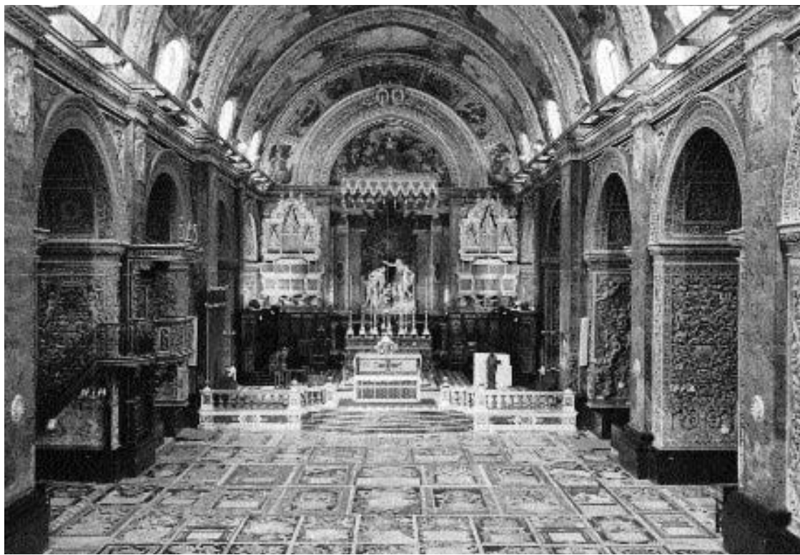
Figure 1.31 St John's Cathedral, Valetta, Malta. Floor entirely covered with ledger stones in coloured marble, mostly dating from the seventeenth century, many to Grand Masters of the Order of the Knights of St John. These fine ledgers are being damaged by stiletto heels, and a conservation programme is in progress (Photograph, Mario Mintoff, Photocity, Valletta)
