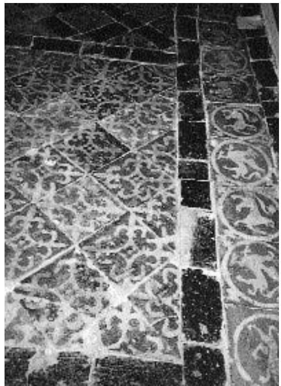
Plate 3 Salisbury Cathedral. Muniment room. Thirteenth-century tiled pavement detail – see page 6 (Photograph, Jane Fawcett)
