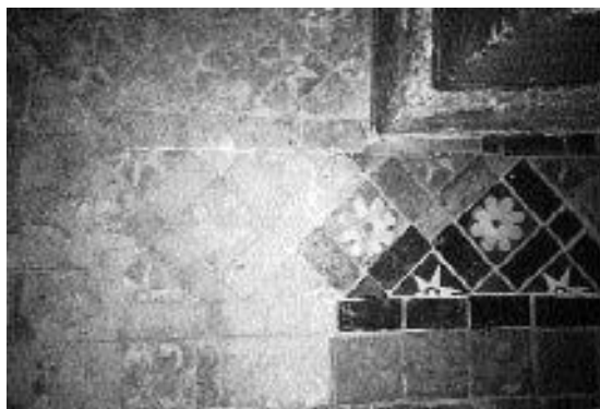
Figure 12.3 Contrasting areas of conserved tiles and replicas and tiles awaiting cleaning (Photograph, Peter Bird)
