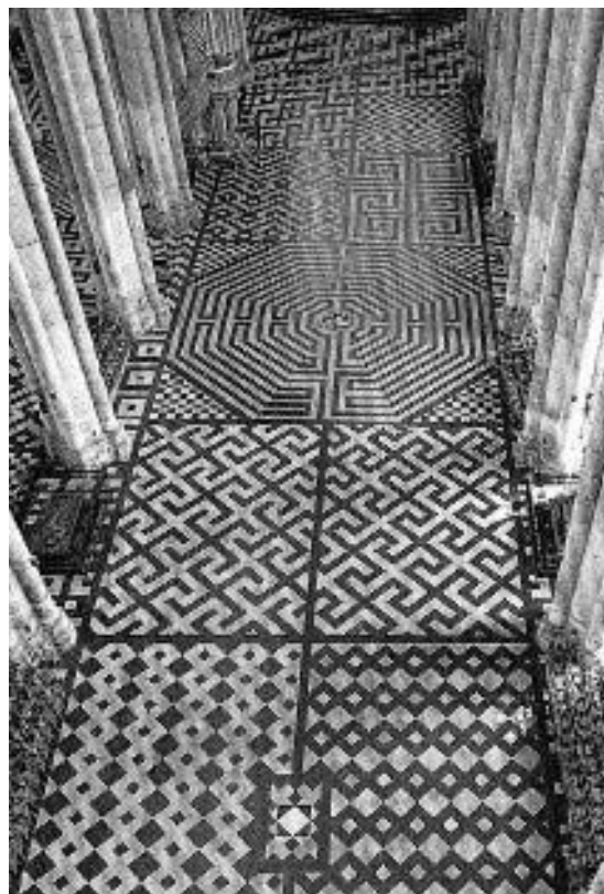
Figure 1.19b Amiens Cathedral, Northern France. Fine marble geometric pavement, containing a representation of a labyrinth, destroyed in 1820 and reinstated in 1894 (By kind permission of the Direction Régionale des Affaires Culturelles de Picardie)
