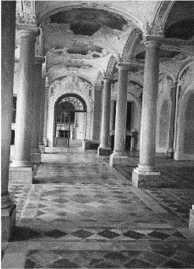
Plate 50 Neues Schloss Schleissheim, near Munich, Germany. Begun in 1701 by Zucalli and decorated in 1715 by Effner, for Max Emmanuel, Elector of Bavaria. The Lower Galley – see page 149 (Photograph, Jane Fawcett)
