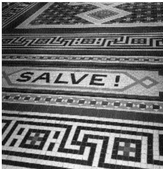
Figure 14.4 Wimpole Hall, Cambridgeshire, c.1793, Soane, and c.1840, Kendall. Encaustic tiled pavement. Entrance hall, c.1840. Kendall (Photograph, Jane Fawcett)
