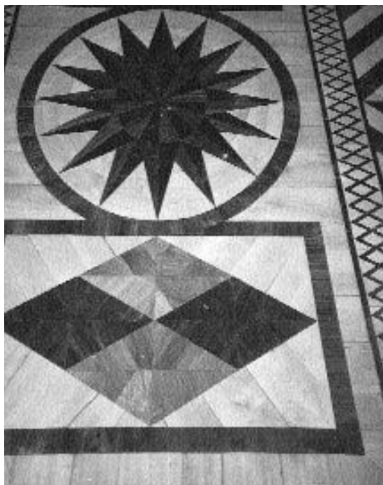
Figure 14.19 Casino, Marino, Dublin, Ireland, 1758–1776. Sir William Chambers. Marquetry floor, restored in the 1980s (Photograph, Jane Fawcett)
