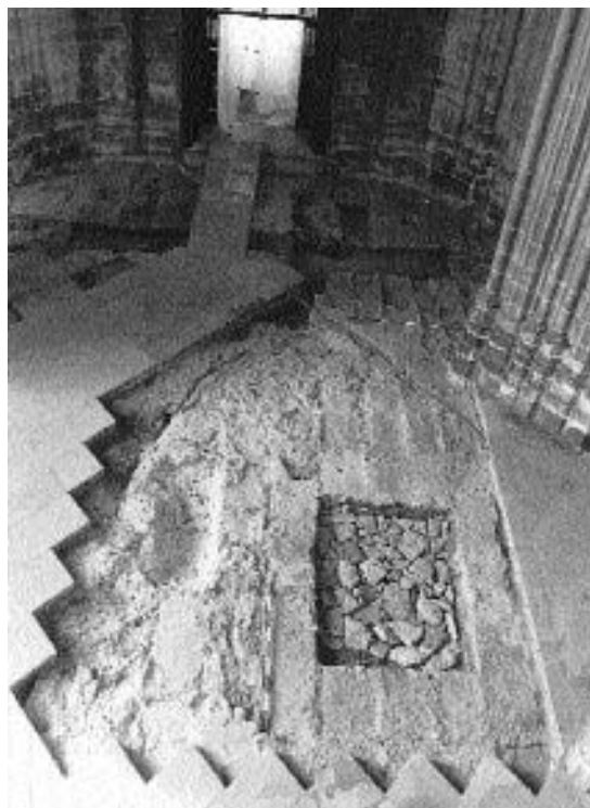
Figure 4.2 Norman floor-bedding mortar at the west end of the nave. Note the broken Norman floor slabs in the backfilled grave (removed during the 1787 reflooring), and the pattern of the 1787 floor slabs (scales 2 m) (Photograph, Canterbury Archaeological Trust)
