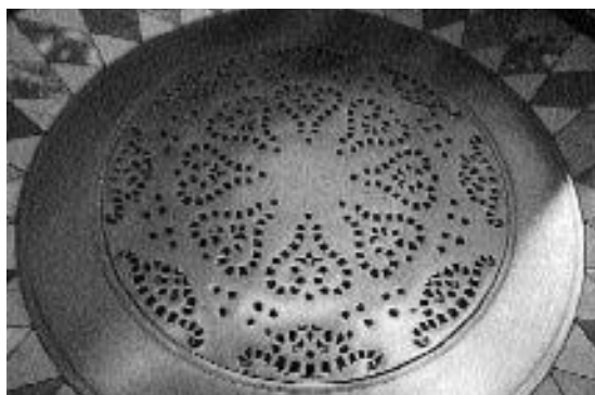
Figure 1.16 St Paul's Cathedral, London. Brass grille with marble surround, central feature of Wren's crossing design (Photograph, Jane Fawcett)
