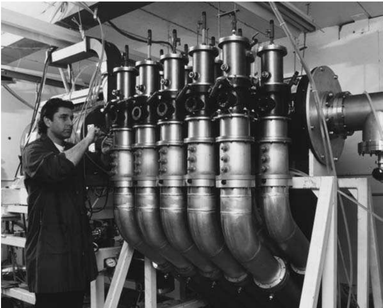
FIGURE 7.22 Inductive adder with 10 pulse-forming lines for the 100-nsec Compact Linear Induction Accelerator. (Courtesy of David Price, L-3 Communications Pulse Sciences.)
