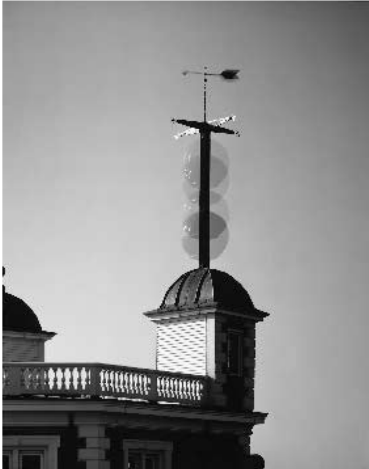
Figure 6.4. The time ball at the Royal Observatory in Greenwich was the world's first regular public time signal. It was dropped at exactly 1 pm every day. This multiple exposure shows the ball at four positions in its journey up and down the mast.
