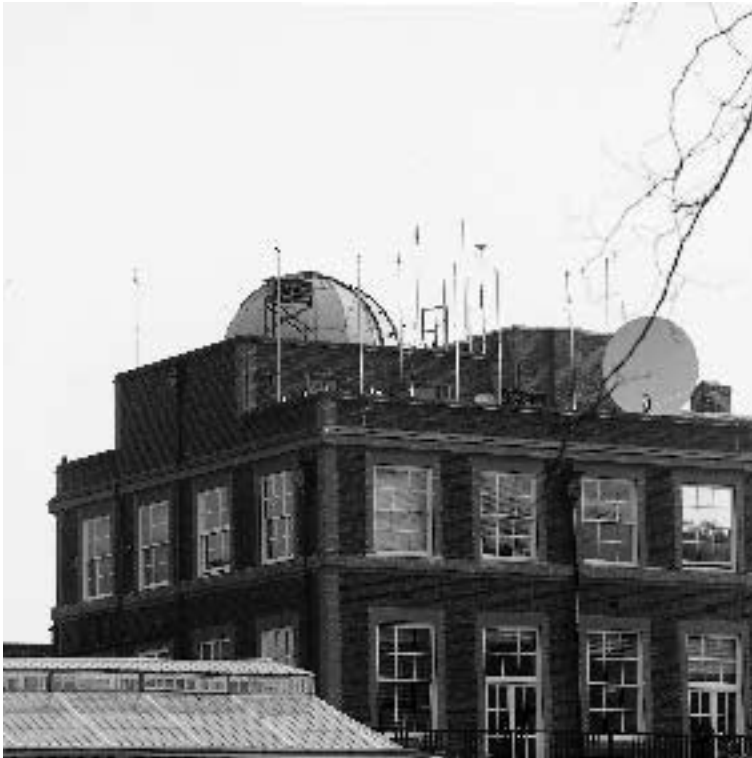
Figure 6.6. An array of GPS receivers being tested on the roof of the time-transfer laboratory at NPL. The dish at the right is for two-way time transfer via geostationary communications satellites.
