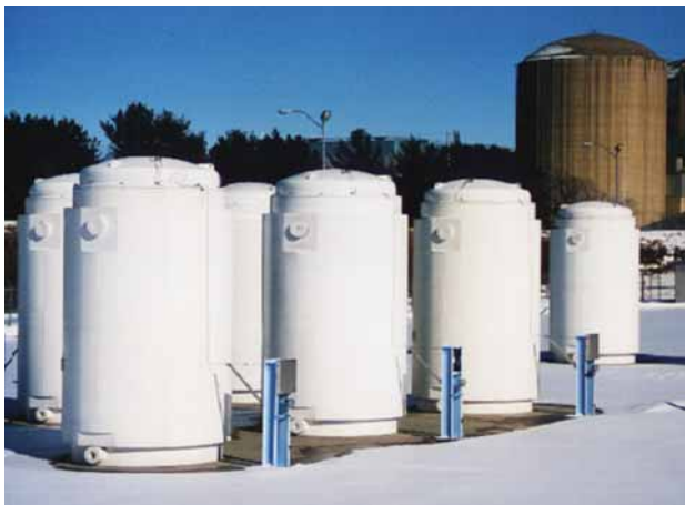
Figure 13-15 Nuclear waste storage. After three or four years in a reactor, spent fuel rods are removed and stored in a deep pool of water contained in a steel-lined concrete basin (left). After they have cooled, the fuel rods are sometimes moved to dry-storage containers made of steel or concrete (right). Question: Do you think these are safe storage methods? Why or why not?
