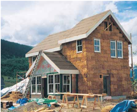
Figure 13-23 Solutions: energy-efficient, environmentally healthy, and affordable Victorian-style straw bale house designed and built by Alison Gannett in Crested Butte, Colorado (USA). The left photo was taken during construction; the right photo shows the completed house. Depending on the thickness of the bales, plastered straw bale walls have an insulating value of R-35 to R-60, compared to R-12 to R-19 in a conventional house. (The R-value is a measure of resistance to heat flow.) Such walls are also great sound insulators. Questions: What are some possible disadvantages of straw bale construction? Do you think they outweigh the advantages? Explain.
