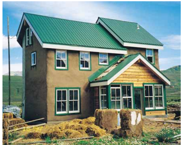
Figure 13-23 Solutions: energy-efficient, environmentally healthy, and affordable Victorian-style straw bale house designed and built by Alison Gannett in Crested Butte, Colorado (USA). The left photo was taken during construction; the right photo shows the completed house. Depending on the thickness of the bales, plastered straw bale walls have an insulating value of R-35 to R-60, compared to R-12 to R-19 in a conventional house. (The R-value is a measure of resistance to heat flow.) Such walls are also great sound insulators. Questions: What are some possible disadvantages of straw bale construction? Do you think they outweigh the advantages? Explain.
