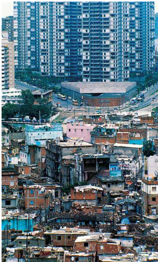
Figure 7-20 Global outlook: extreme poverty forces hundreds of millions of people to live in slums and shantytowns such as this one in Rio de Janeiro, Brazil, where adequate water supplies, sewage disposal, and other services do not exist.
