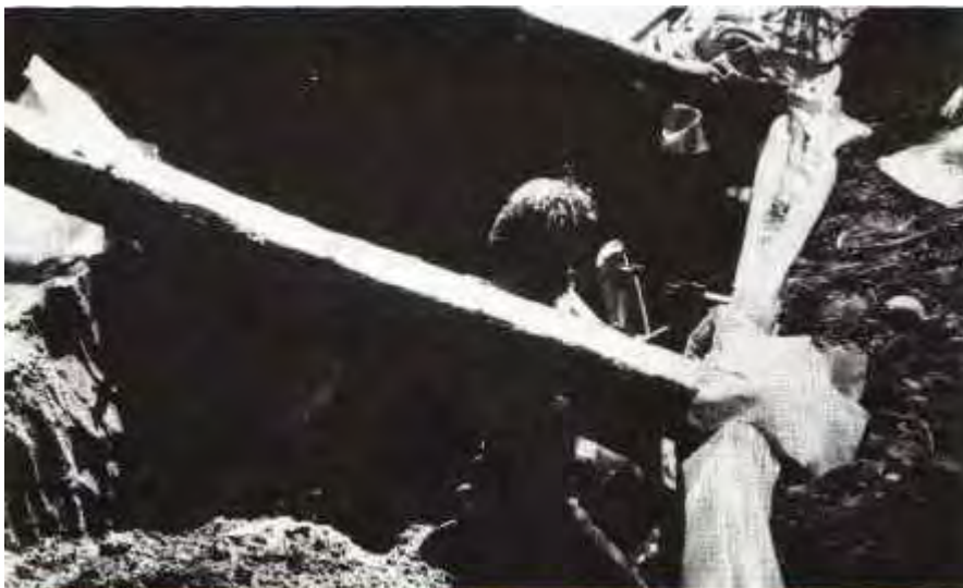
Left: Mike begins work on the lower wall of the $50 house.
