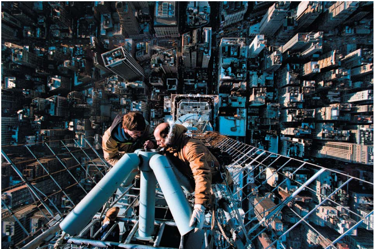
Workers repair the antenna atop the Empire State Building in 2001.
