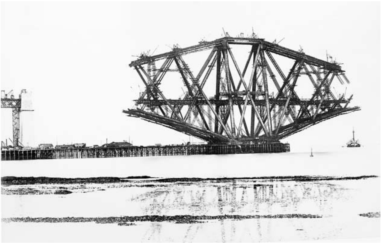
Figure 2.4 Black-and-white film is the ideal medium for the archival recording of buildings, having proved its durability over a long period of time, and is more consistent than colour for the direct comparison of shots. This photograph was taken at the turn of the century by William Dunn (great-grandfather of the author) of the Forth Railway Bridge in Scotland under construction
