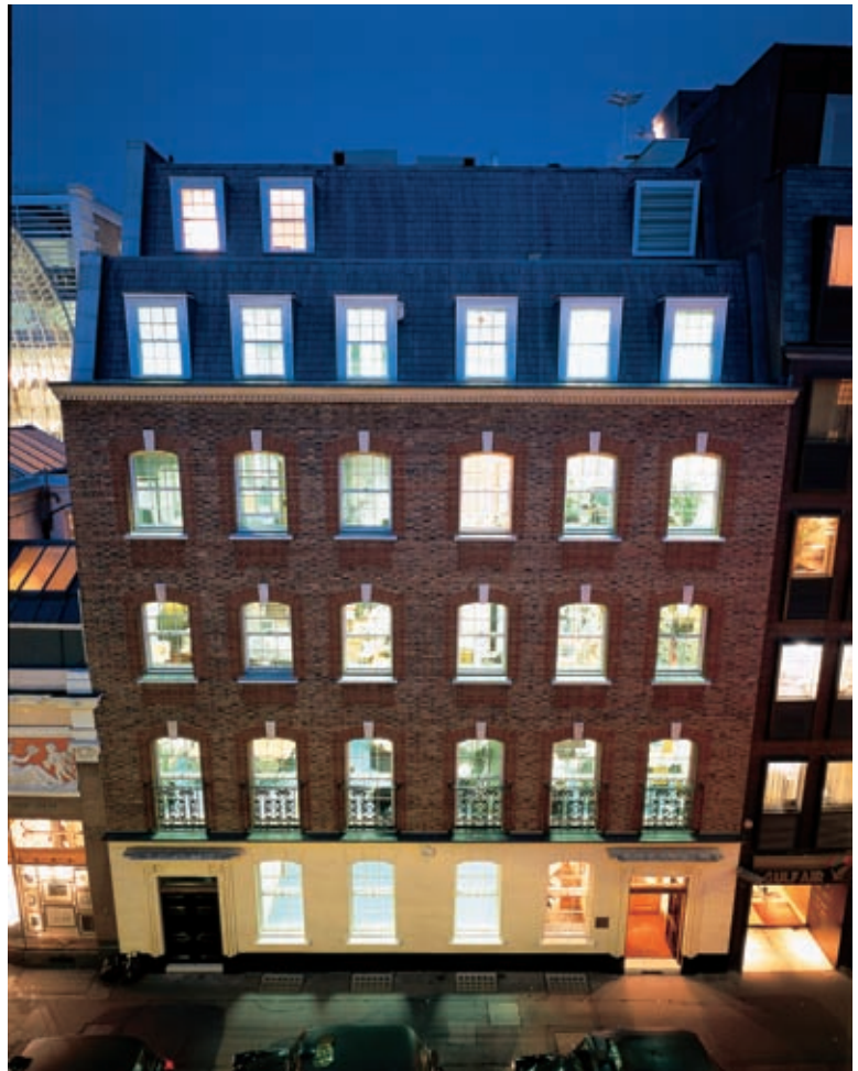
Figure 8.7 A typical night shot, actually taken at dusk. The sky retains sufficient brightness for the outline of the building to be satisfactorily silhouetted and detail of the structure to be just visible. Uniformity of the interior lighting is essential for such shots
