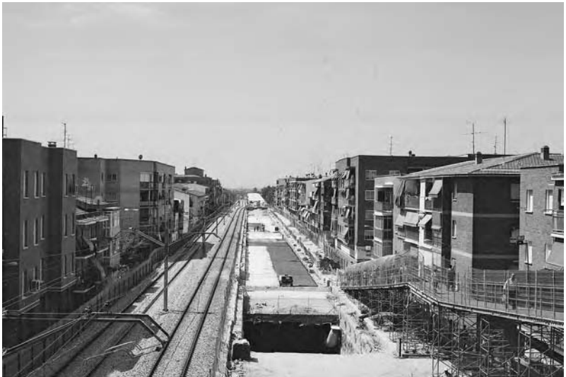
Figure 5.3 The burying of the suburban railway line
