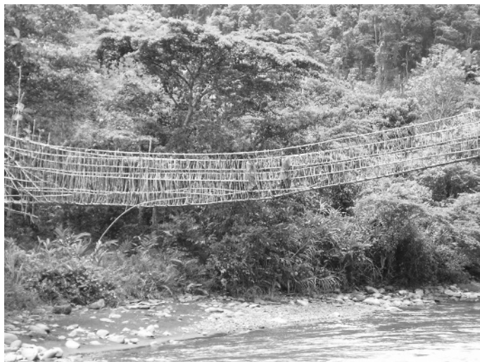
FIGURE 3.23 Lashed pole suspension bridge over the Fu River, Papua New Guinea.
