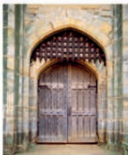
GATEHOUSE The main entrance was often fortified by a movable iron grate called a portcullis.
