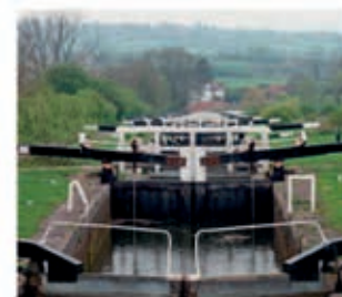
CAEN HILL LOCKS A series of 29 locks on the Kennet and Avon Canal in England were built in 1810 by John Rennie.
