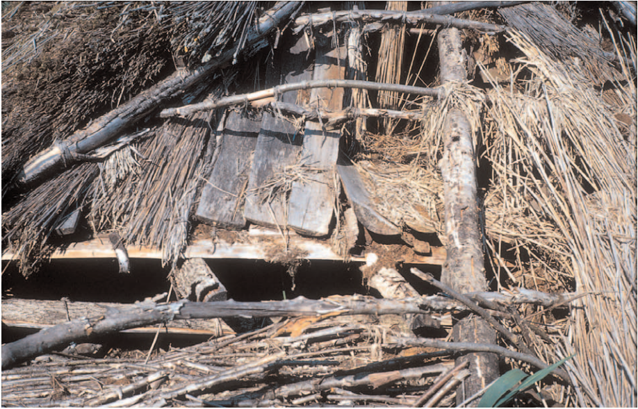
Figure 16.2 The Neolithic house from Chalain, France, reconstructed by the Centre de Recherche Archéologique de la Vallée de l'Ain fell on to the ground in 2002 and was left untouched where it fell, so one can still see how it was built. The construction is deliberately being left to decay. The floor, which was originally 1.2 m above the ground, collapsed, but remained intact in 2002. Photograph: Urs Leuzinger, Archaeological Department, Canton, Thurgau.
