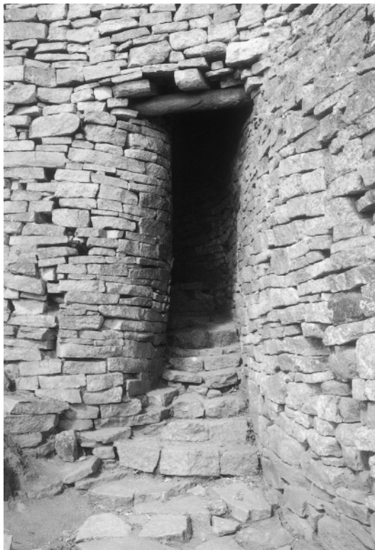
Figure 62 A stepped doorway in the hill-ruin at Great Zimbabwe. The curved stonework is characteristic.
