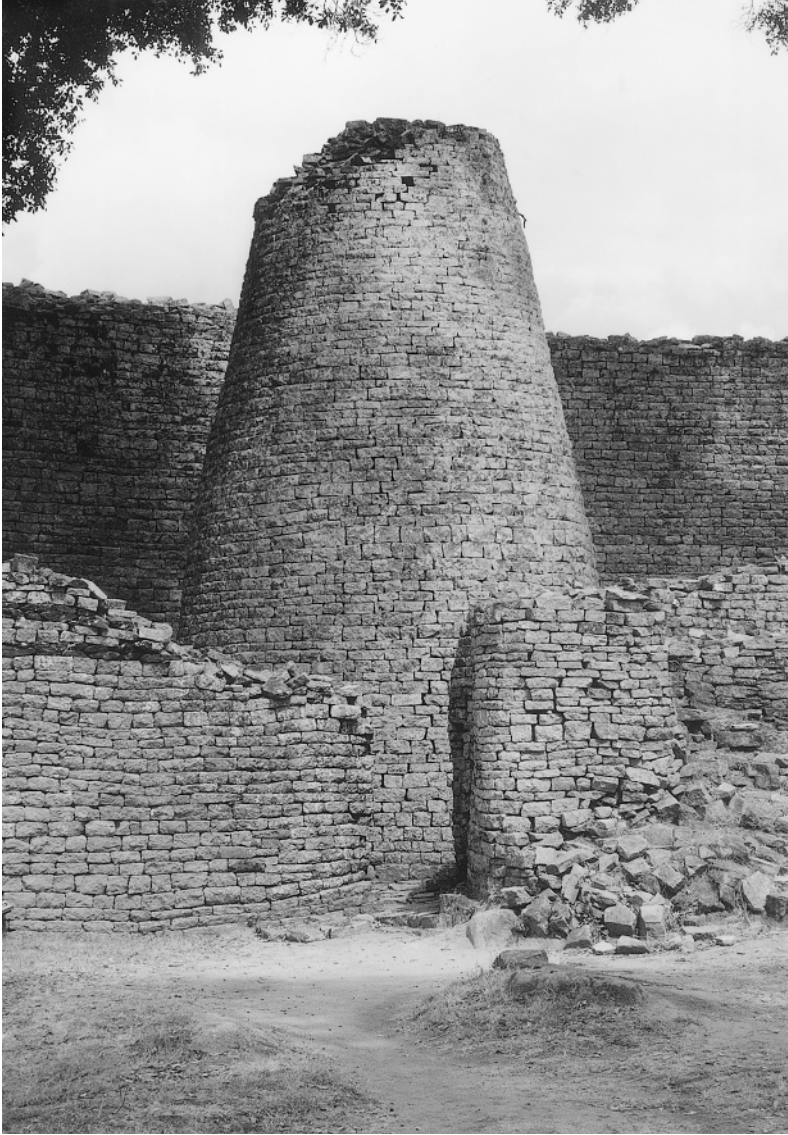
Figure 61 The conical tower in the large valley enclosure at Great Zimbabwe. Over 9 metres high, it shows a remarkable mastery of drystone masonry technique.
