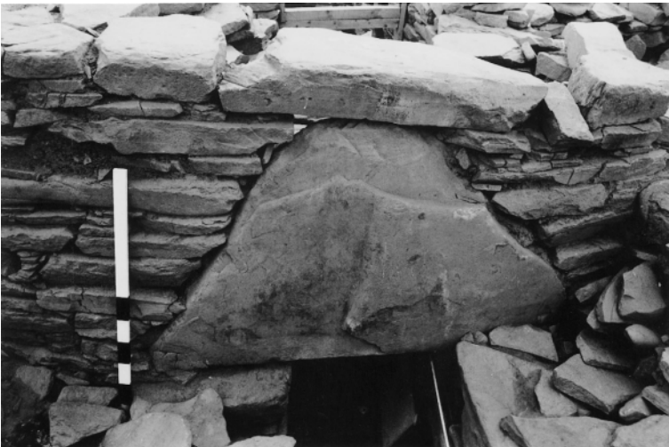
Figure 5.5 (opposite and above) Complex Atlantic roundhouses with triangular entrance lintels. 1 (opposite), Culswick, Shetland; 2, Dun Dornadilla, Sutherland; 3, Old Scatness, Shetland. Photographs by D. W. Harding and I. M. Blake.
