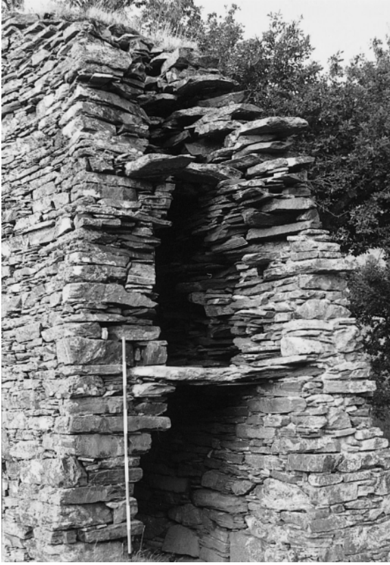
Figure 5.4 Dun Troddan, Glenelg, Inverness-shire, showing stonework of intra-mural gallery. Photograph by D. W. Harding.
