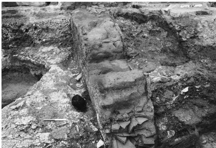
Figure 43 Early second-century clay block wall from Watling Court, London. Copyright Museum of London.
