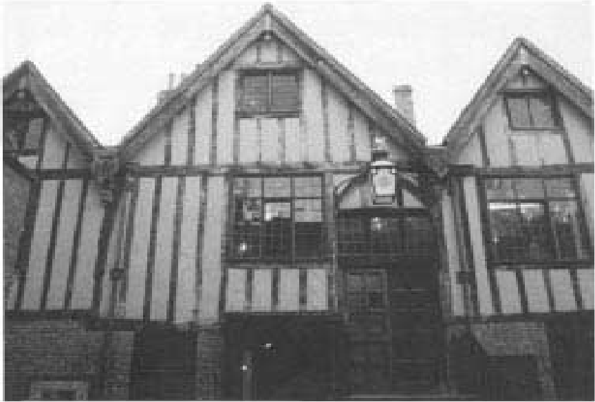
Figure 6.4 Exterior of the north-east range, Trinity Hall (the Merchant Adventurers' Hall), York
