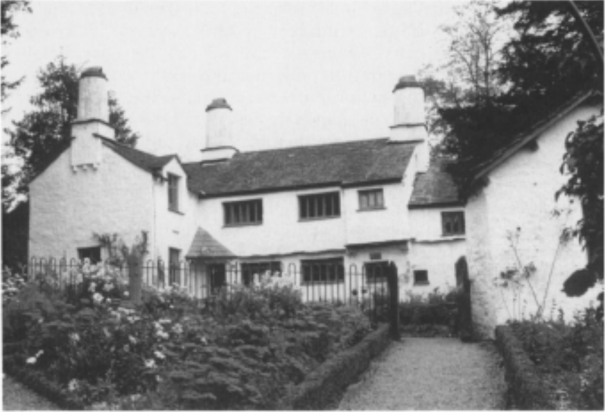
50 Townsend, Troutbeck, Cumberland, a remarkably well-preserved example of a prosperous Lake District yeoman farmer's house, built of stone with oak mullioned windows. The central, recessed block dates from the late sixteenth century. The wing on the right containing the kitchen was added in about 1623. The projecting wing on the extreme right is a dairy added in the nineteenth century. The wing on the left was added in the eighteenth century.
