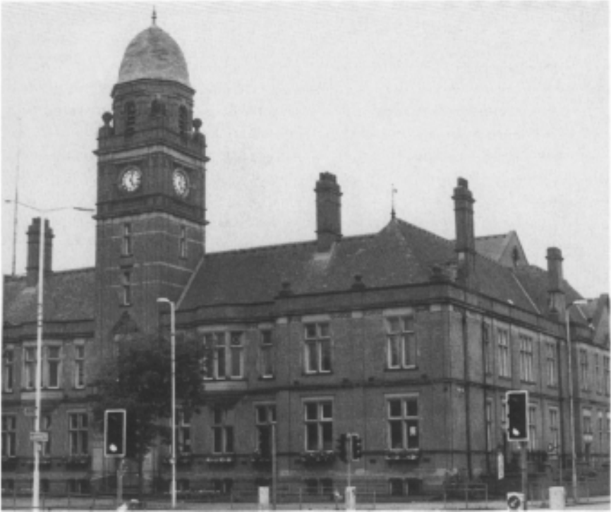
81 The town hall at Hyde, Cheshire, built between 1883 and 1885 to designs by J.W.Beaumont.
