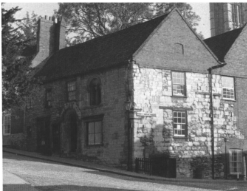
32 Aaron the Jew's House, Lincoln, a stone town house built in the late twelfth century.
