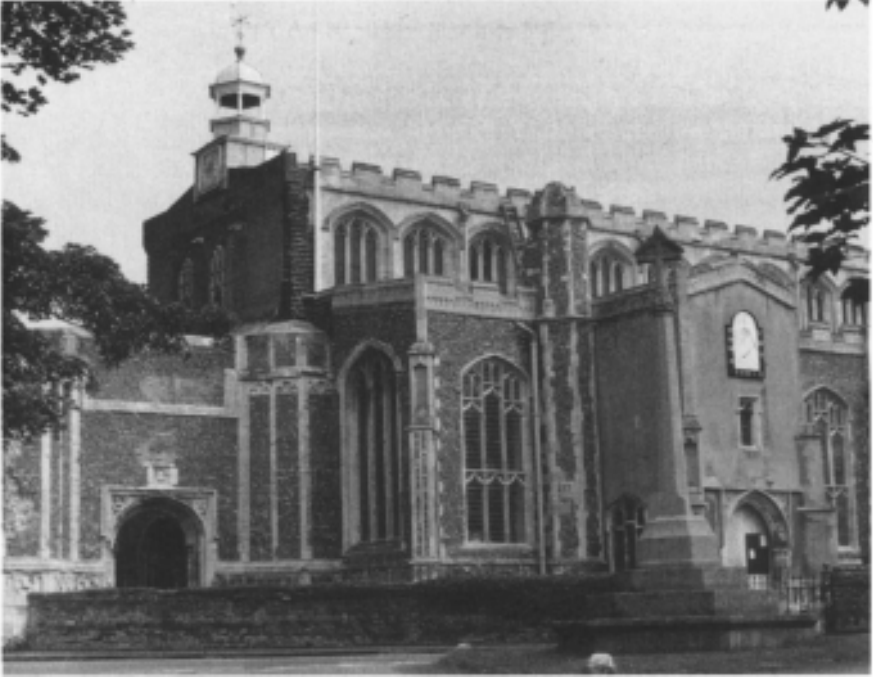
40 The church at East Bergholt, built partly of brick and partly of flint in the late fifteenth century. The west tower was begun in 1525 but never finished.
