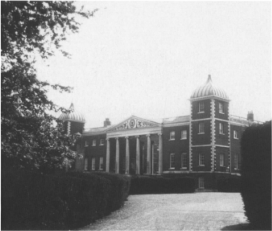
65 Osterley Park, Middlesex. The original house was built by Sir Thomas Gresham in the 1570s. It was then remodelled by Robert Adam, who added the splendid portico, finished in about 1773, as a screen across the mouth of the courtyard to the original house.
