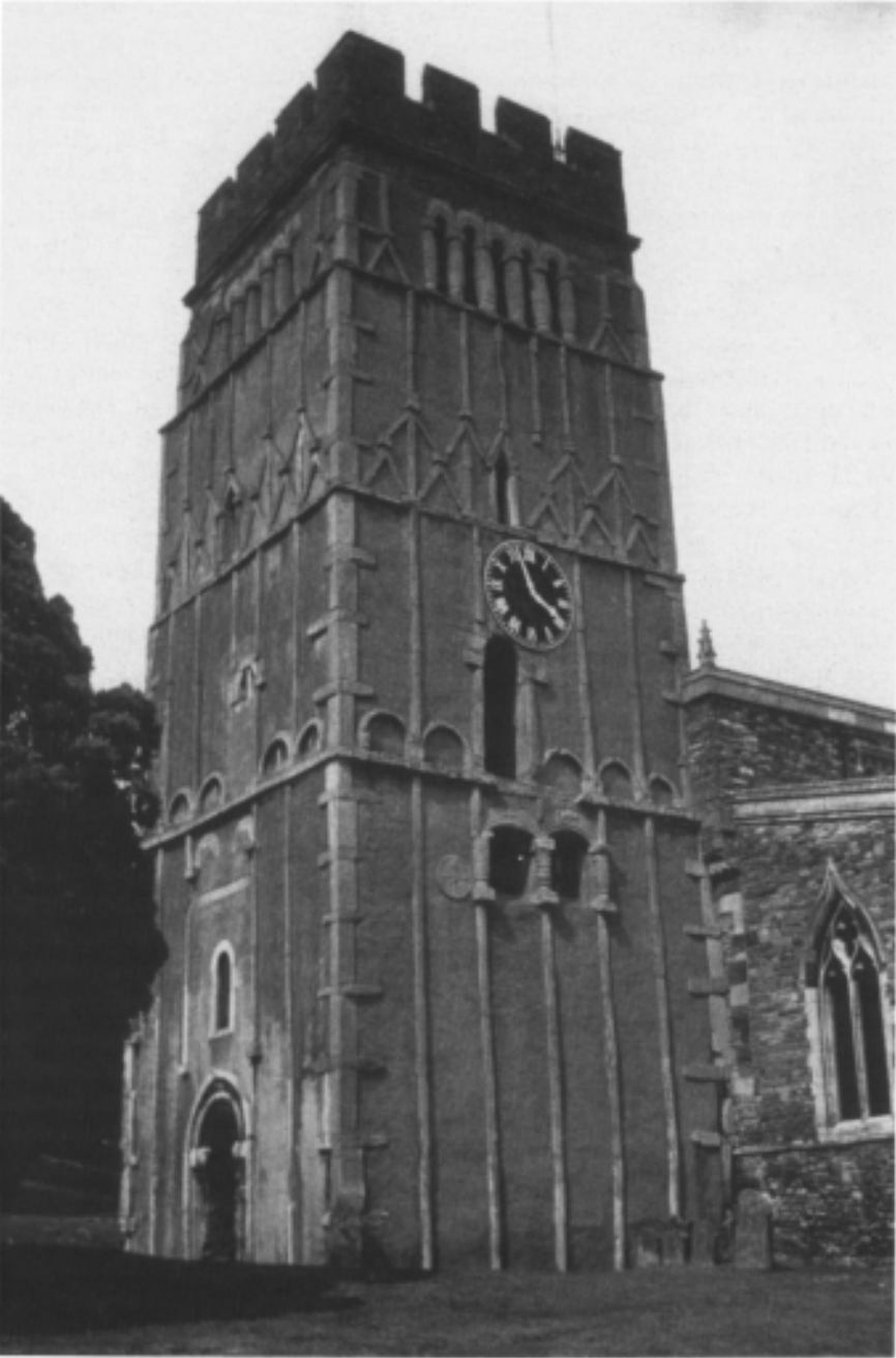
36 The west tower to the church at Earls Barton in Northamptonshire, built very late in the tenth century. Among its most striking features are the long and short quoining, the strip pilasters, the monumental doorway, and the unusual belfry window openings.
