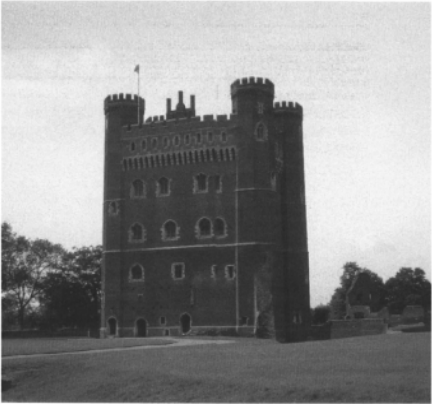
28 Tattershall Castle, Lincolnshire. A castle was first built here in 1231, but this splendid keep, begun in 1434, was built in brick by Ralph Cromwell, Lord Treasurer of England. It stands within a double moat.
