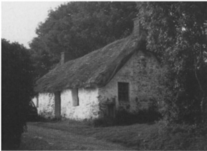
51 A cottage at Torthorwald, Dumfriesshire. Built late in the eighteenth century, it is the last surviving example of a long tradition of cruck building in southwestern Scotland. There are three pairs of internal oak trusses, and the roof is thatched.
