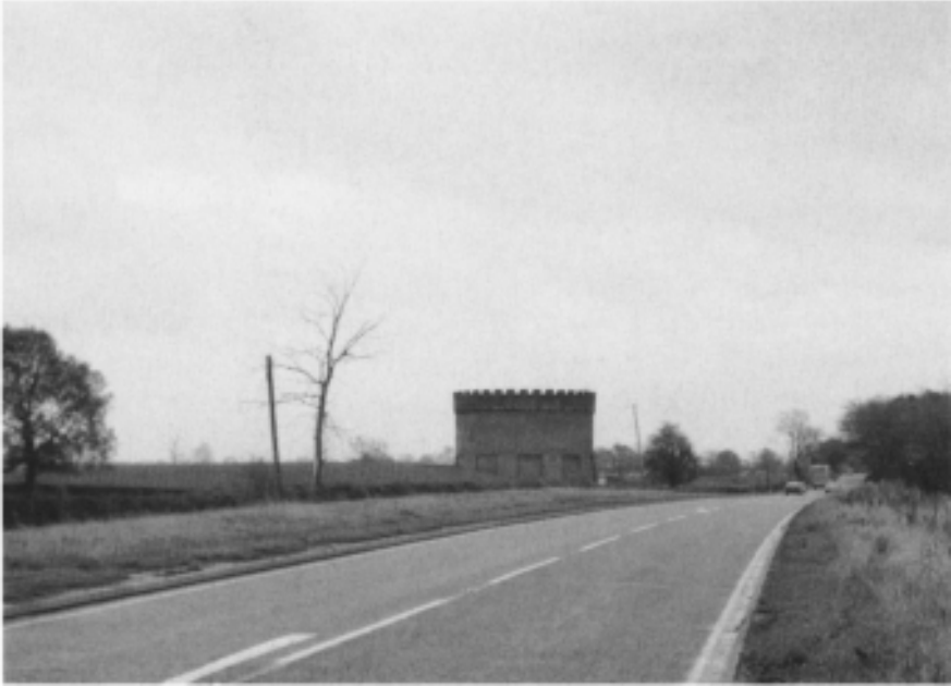
90 A ventilation shaft to the Kilsby Tunnel, Northamptonshire, 1 mile and 682 yards long and built in 1838.
