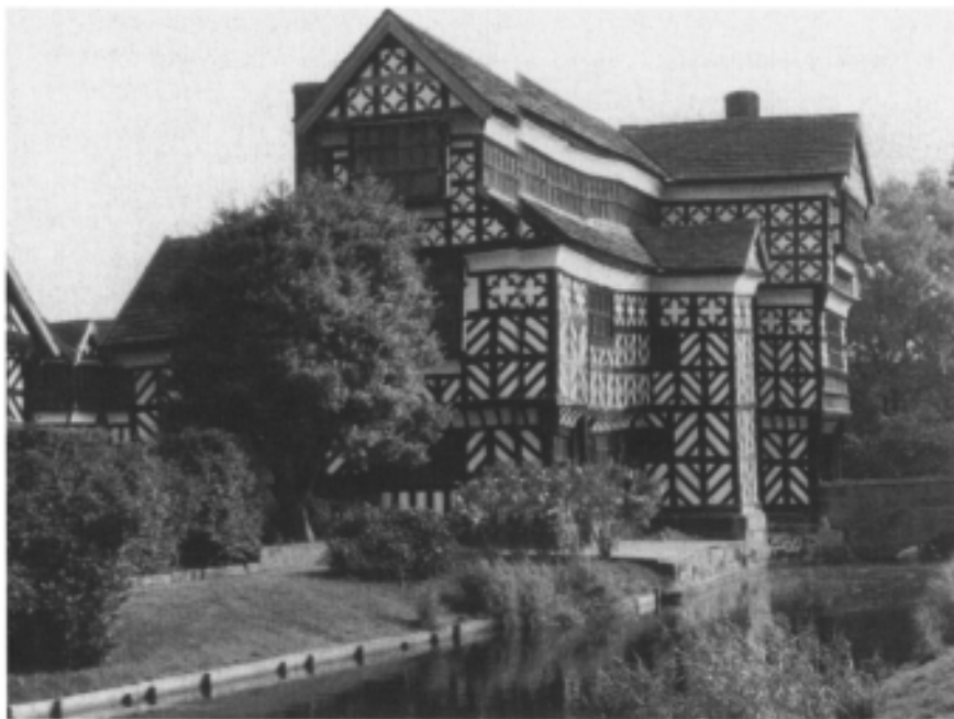
26 Little Moreton Hall, Cheshire, a splendid timber-framed moated house built between the end of the fifteenth and the end of the sixteenth centuries.
