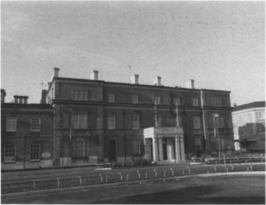
92 Derby Midland Hotel, built in 1840 and the first railway hotel in Britain.
