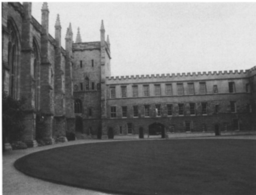
48 New College, Oxford. The Great Quad. On the immediate left is the Chapel, and then the first floor hall, entrance to which is through the door in the Muniment Tower in the corner. The ranges of buildings about the Quad had a third storey and battlements added in 1674 and the windows had sashes inserted in about 1718.
