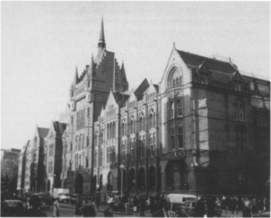
80 The Prudential building, Holborn, built to designs by Alfred Waterhouse between 1899 and 1906 on the site of Furnival's Inn.
