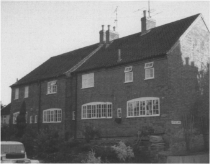
72 Stocking-frame knitters' cottages at Calverton, Nottinghamshire, built in the first half of the nineteenth century. They have long windows on the ground floor in order to give as much light as possible to the machinery.
