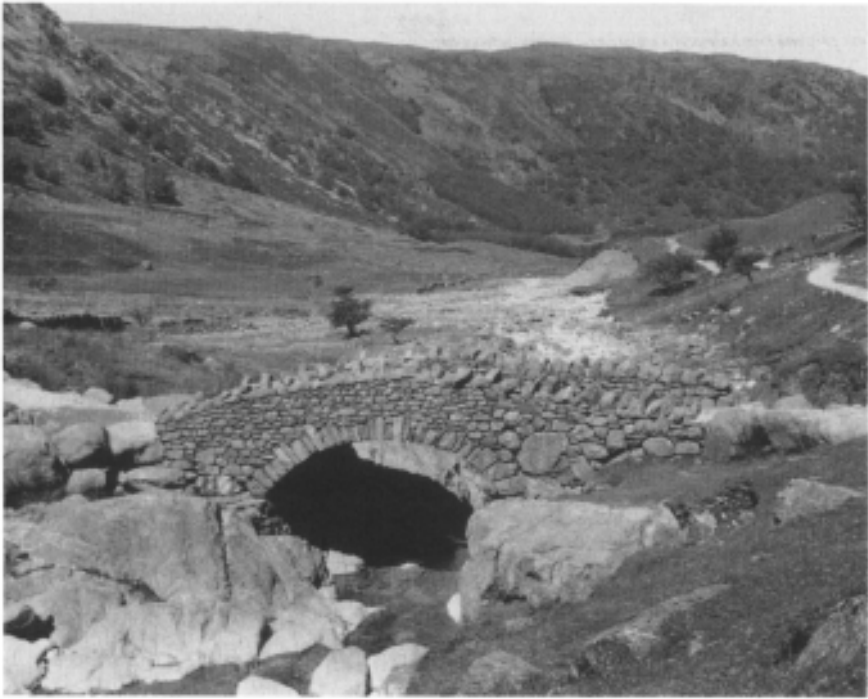
75 Stockley Bridge, Cumberland, a stone packhorse bridge of uncertain date.
