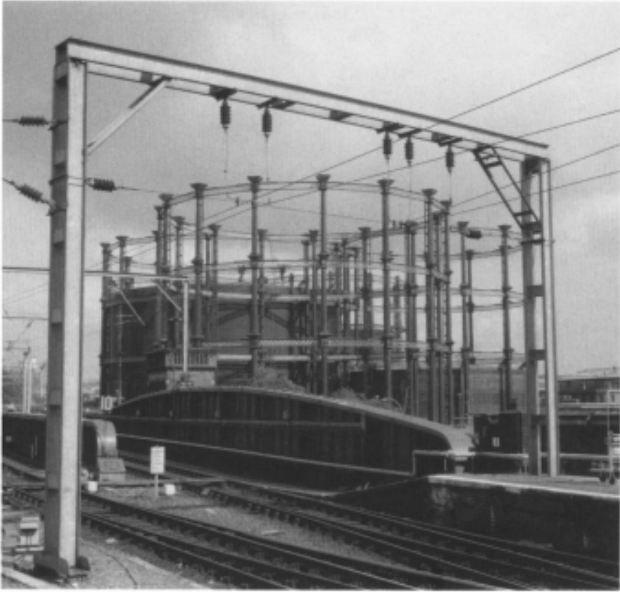
82 The gas holders just outside St Pancras Station, London.
