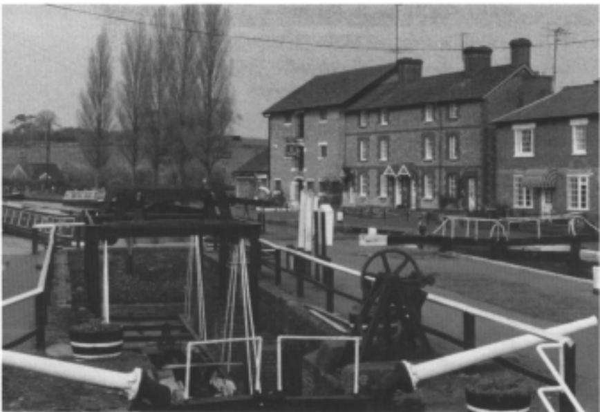
77 Canal locks and wharves at Stoke Bruerne, Northamptonshire, built for the Grand Junction Canal just to the south of the Blisworth Tunnel which, when opened in 1805, completed a waterway link between London and the midlands.
