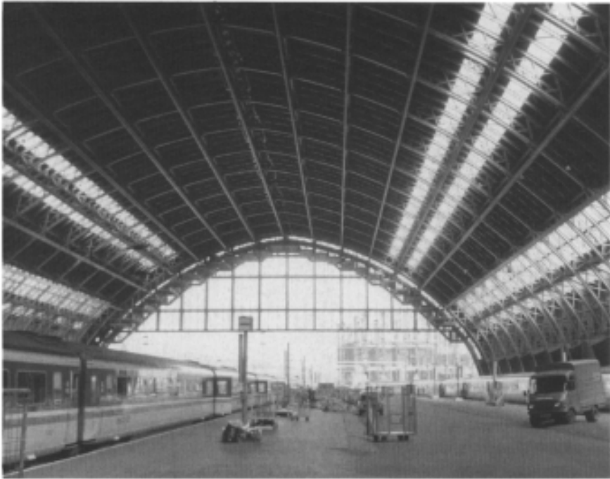
91 The magnificent roof to St Pancras Station, London, built in 1868, the ironwork being manufactured by the Butterley Iron Company.
