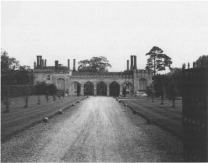
66 Nether Winchendon House, Buckinghamshire, an early sixteenth-century house Gothicized at the very end of the eighteenth century when the screen and battlements were added.
