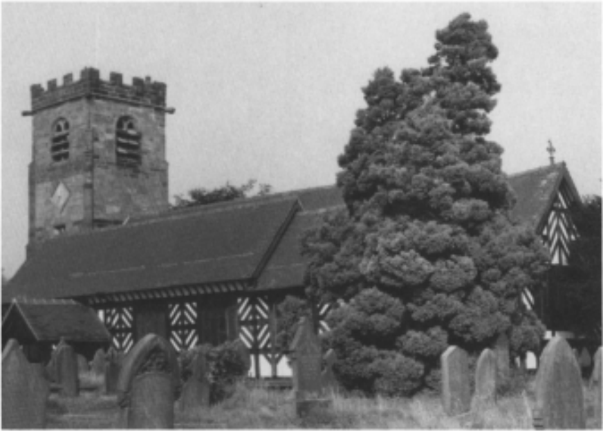
39 Little Peover Church, Cheshire, a fourteenth-century timber-framed church, although much restored.
