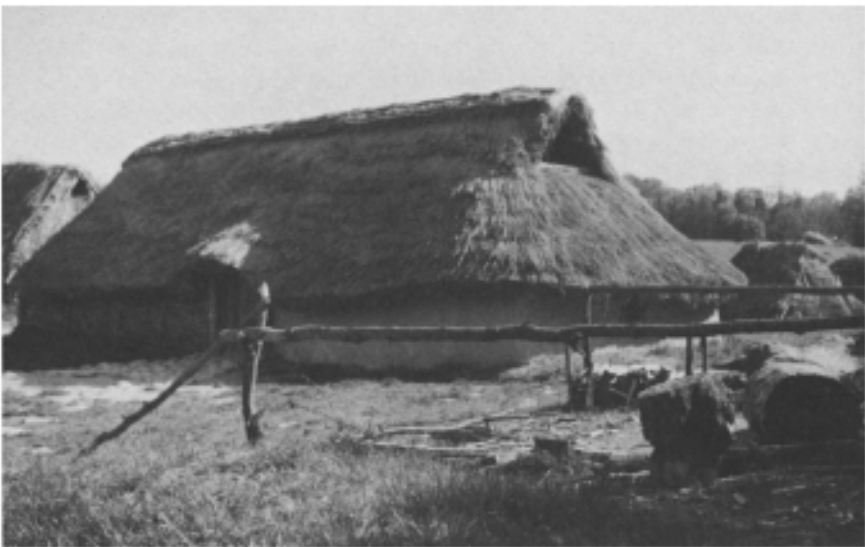
Figure 64 Reconstruction of the typical three-aisled Early Iron-Age house at the Historical Archaeological Experimental Centre at Lejre, outside of Copenhagen.
