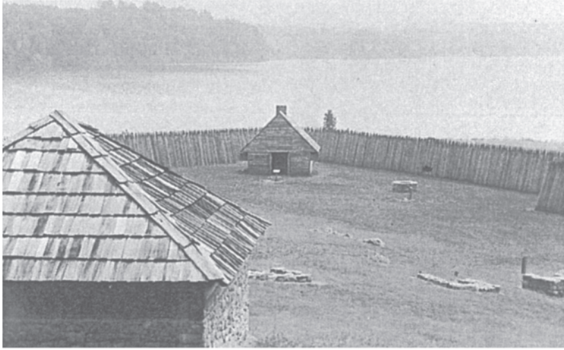
Figure 21.6 A view in a south-westerly direction across the reconstructed fort. The powder magazine is in the left foreground, and the blacksmith's shop is in the distance.
