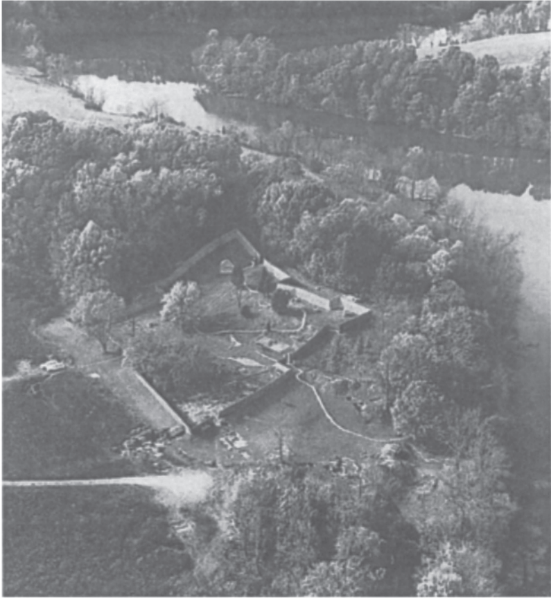
Figure 21.4 An oblique aerial view of Fort Loudoun, taken in 1975 after the beginning of the 1975 excavations. The photograph shows the location of the fort on a narrow ridge adjacent to the Little Tennessee River. The reconstruction of the palisade dates from the 1960s. (Photograph courtesy of Tennessee Valley Authority.)
