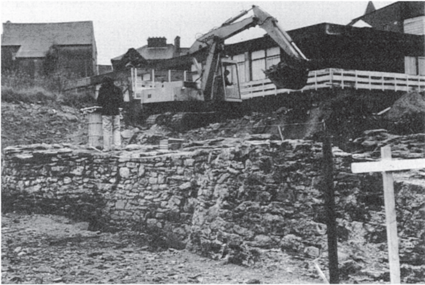
Plate 15 The base of St Martin's Gate, Waterford
