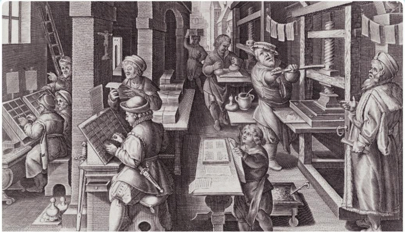
A printing press (on the right) in a printer's workshop.
