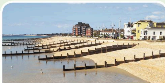
Groynes reduce the force of the waves on the beach and help to make the beach larger.
