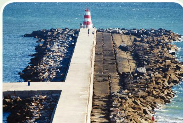
Large lumps of rock have been placed in front of this breakwater in Portugal to break up the force of the waves.
