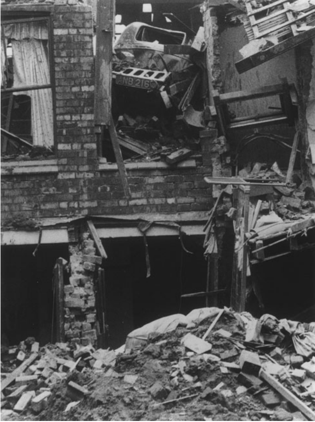
Fig. 5.23 ( left ). Manchester air raid damage.
