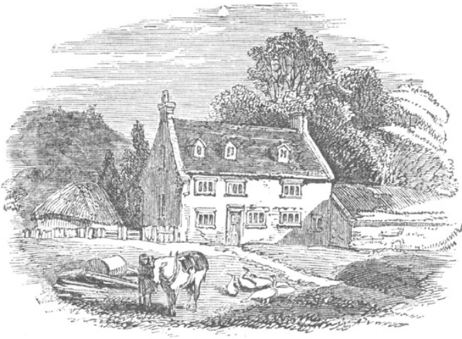
FIG. 3.1. Woolsthorpe Manor, where Newton grew up. It appeared much the same in a sketch dated 1721 and reproduced by Stukeley (1936). According to the latter's Memoirs of Sir Isaac Newton's Life , it had become 'much decay'd' and was re-built by Newton's stepfather, Rev Barnabas Smith, soon after Newton's birth (from Mitchell 1856).
