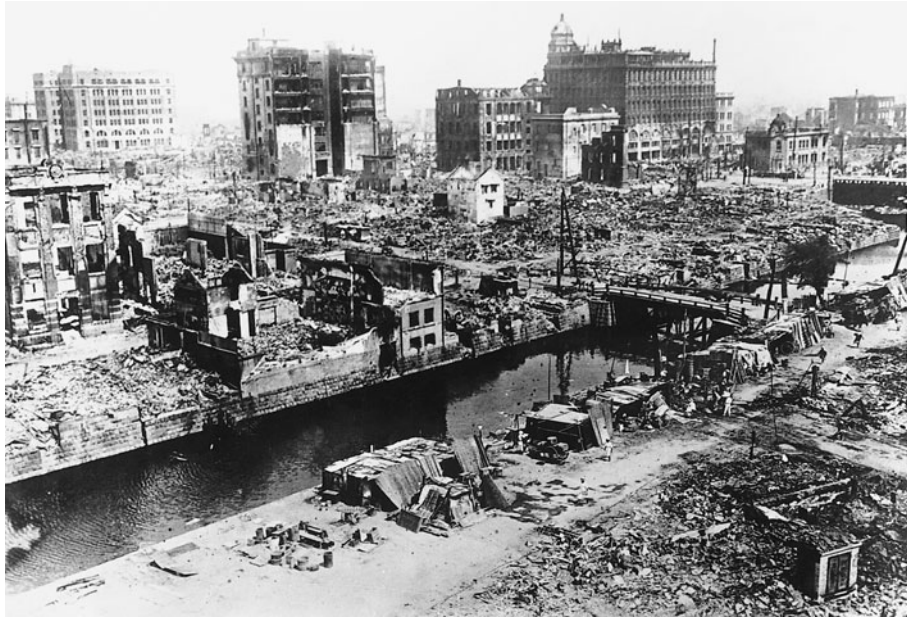
16. Little remained standing after the post-quake fires had raged for two days across Tokyo following the Great Kanto Earthquake of 1923
