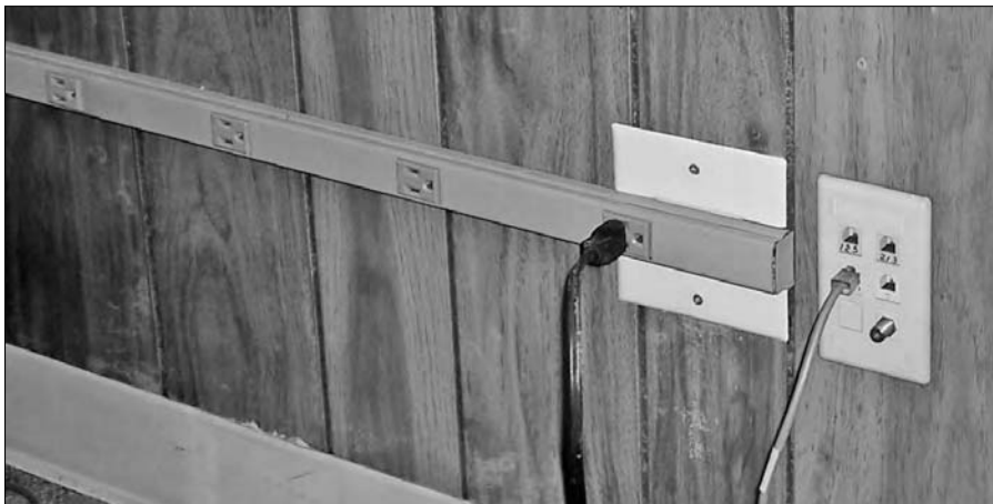
Figure 3-5: This Wiremold outlet strip can be mounted under the kitchen's upper cabinets.
