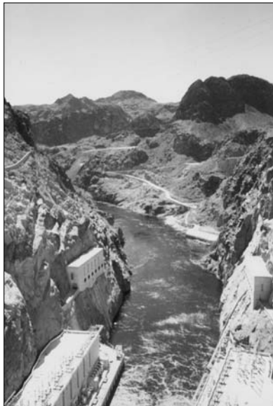
Figure 5-4: The movement of water flows closely along one line and ends at an intersection.
