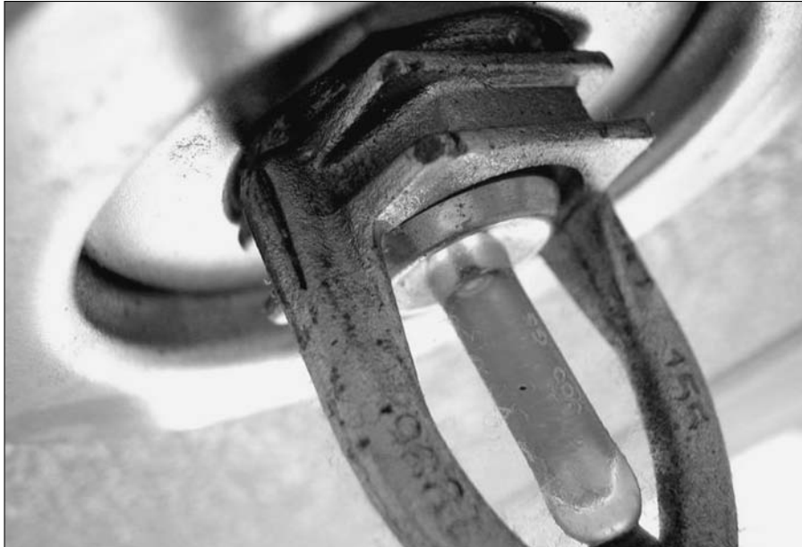
Figure 6-11: The link capsule in a sprinkler head.
