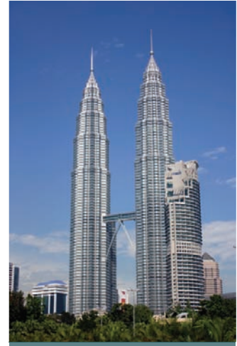
The Petronas Twin Towers in Kuala Lumpur look congruent.
