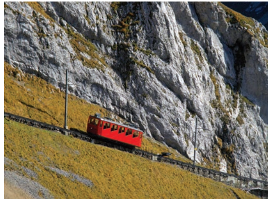
The slope of this mountain railway could be expressed in the form y = mx + c .
