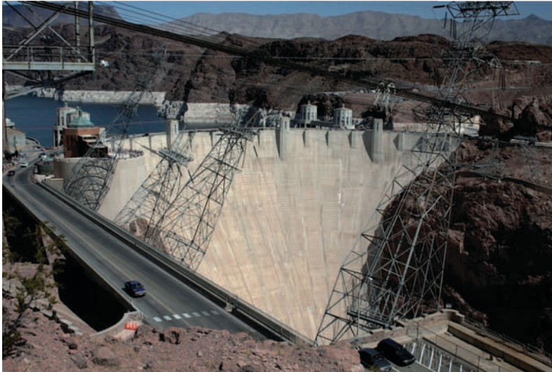
At the time of construction, the Hoover Dam was the largest concrete structure in the world.
