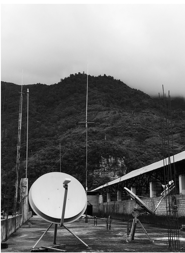
Figure 22.1 Antennas and dead infrastructures of Nuyoo.
