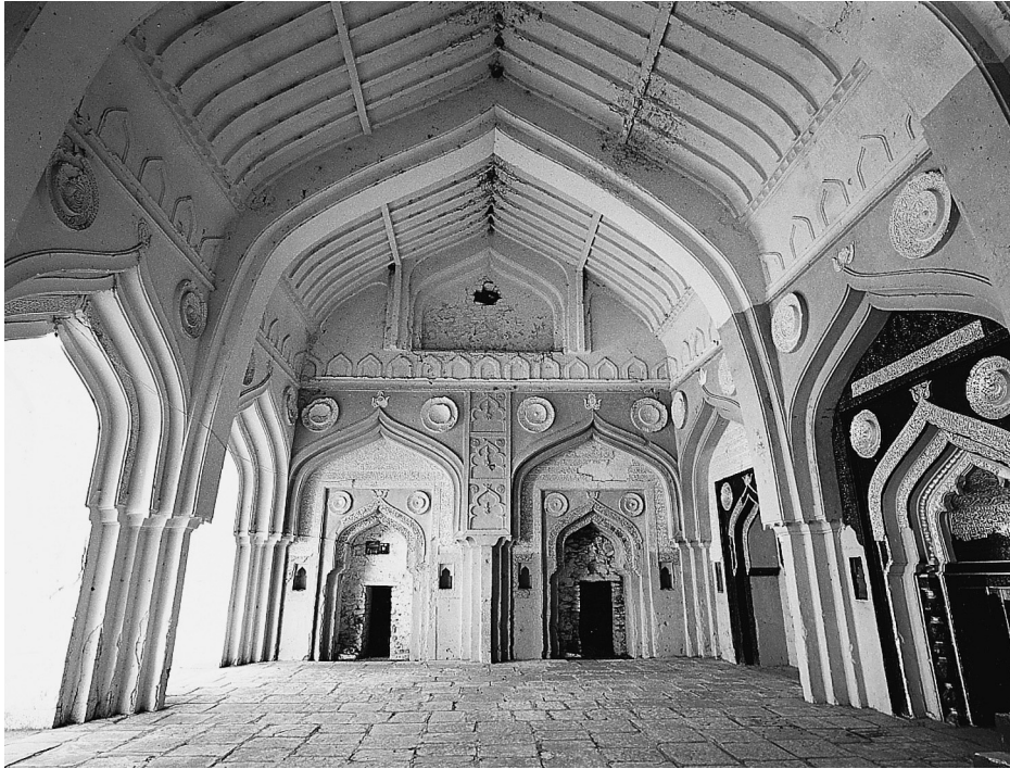
42 Interior of Langar-ki mosque, Gulbarga, fifteenth century
