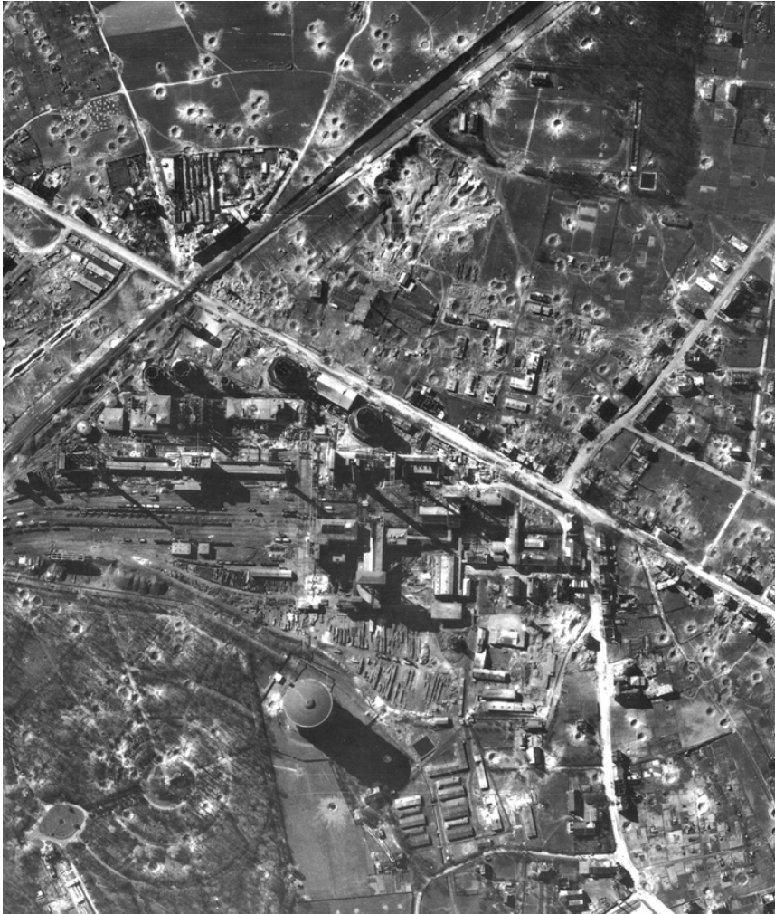
Fig. 3.1-3: World War II aerial photograph (March 24, 1945) of a destroyed industrial complex in the Dortmund area (Ruhr district, Germany). Damaged industrial plants, from which pollutants may have seeped into the soil, and bomb craters and pits, which may have served as dumps, are potential hazardous sites (courtesy of Luftbild-Datenbank, Ing.-Büro Dr. Carls, Estenfeld).
