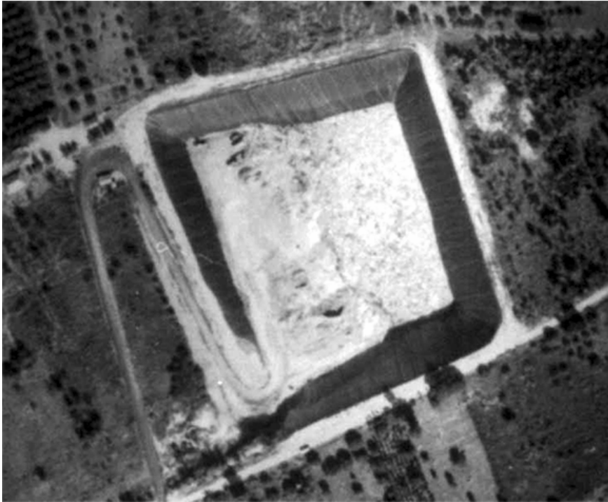
Fig. 3.1-1: Black-and-white aerial photograph taken by the Royal Thai Survey Department on November 11, 1995, showing the more than 35 m deep Nong Harn borrow pit near Chiang Mai in northern Thailand. The pit is being filled with waste from the west along a road to the bottom of the pit. The pit has steep slopes and was previously about 45 - 50 m deep. The western part of the pit floor is covered by more than 10 m of waste. The southern, western, and eastern slopes are covered by a plastic liner. The fine white lines on these slopes are ropes to hold down the strips of the liners. The northern slopes have the ropes too, but no plastic liner cover, as indicated by the brighter gray color and by the micro-topography of the uncovered slope.
