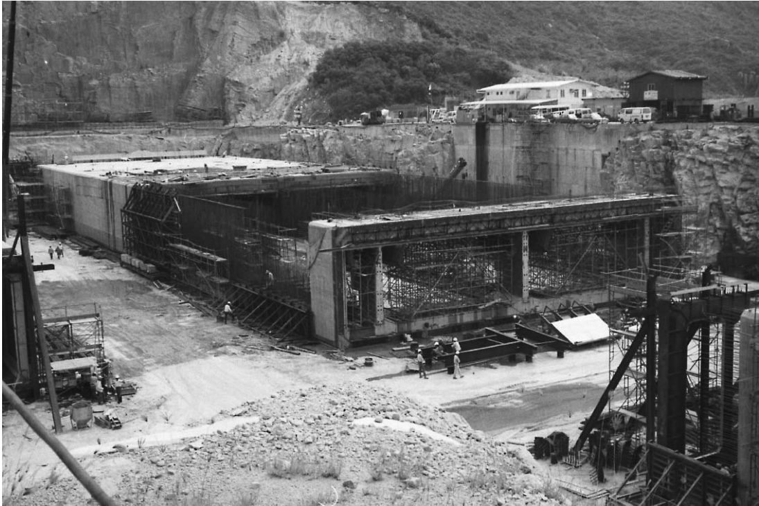
Fig. 20.24 Western Harbour Crossing, Hong kong.
