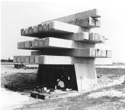
Fig. 7.23 Static-load test on a pile with dead weight as the reaction load.
