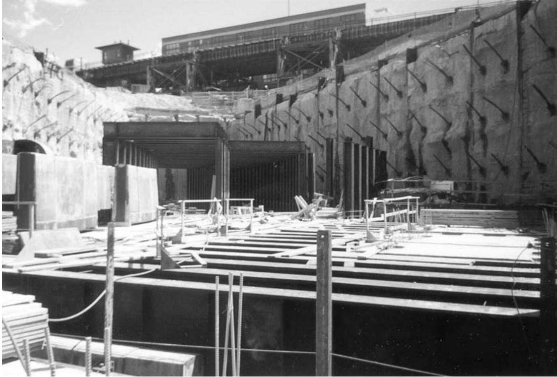
Fig. 20.8 63rd Street Tunnel Strutting and Tie-backs.
