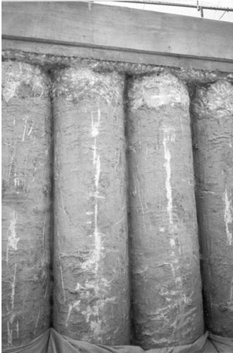
Fig. 20.9 Tangent Piles.
