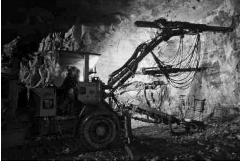
Fig. 20.10 Drill and Blast (TARP).
