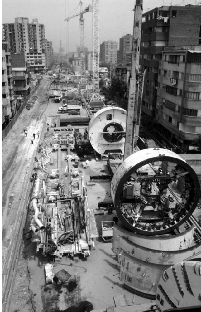
Fig. 20.21 Preparing the Cairo Metro Shield for Assembly.
