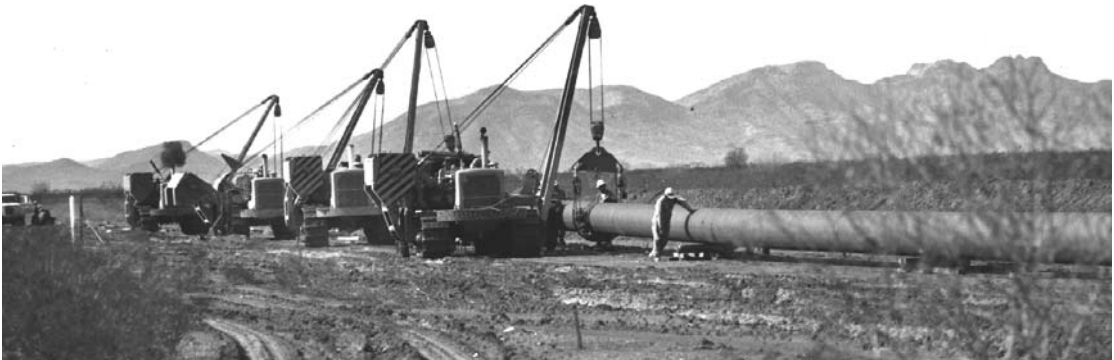
Fig. 13.11 Pipelayers. ( Caterpillar Tractor Co. )
