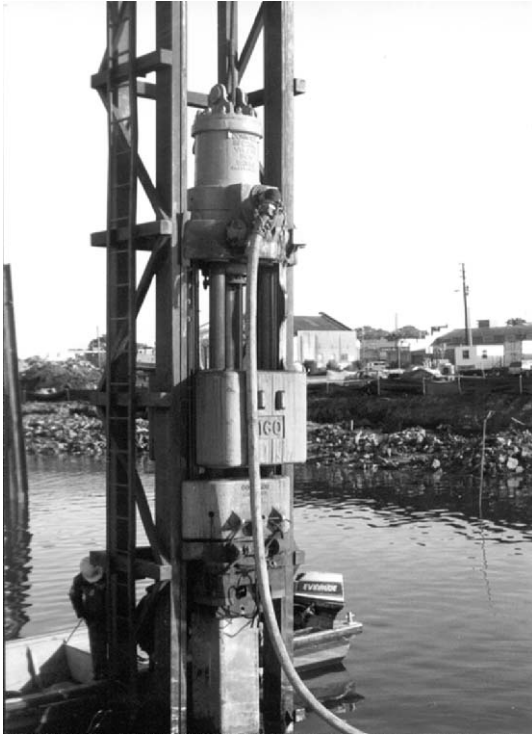
Fig. 7.18 Single-acting, external-combustion hammer driving a precast concrete pile.
