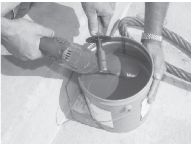
Figure 3-25: Epoxy grout being mixed
