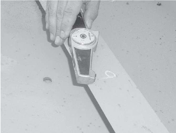
Figure 3-18: Verification of coating thickness is important
