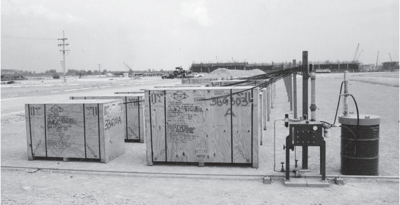
Figure 10-21: Crated oil mist-protected outdoor equipment storage in a hot and humid Gulf Coast environment. Oil mist header, distribution manifolds and oil mist generator are shown to the right of picture. (Source: Lubrication Systems Company, Houston, Texas 77024)
