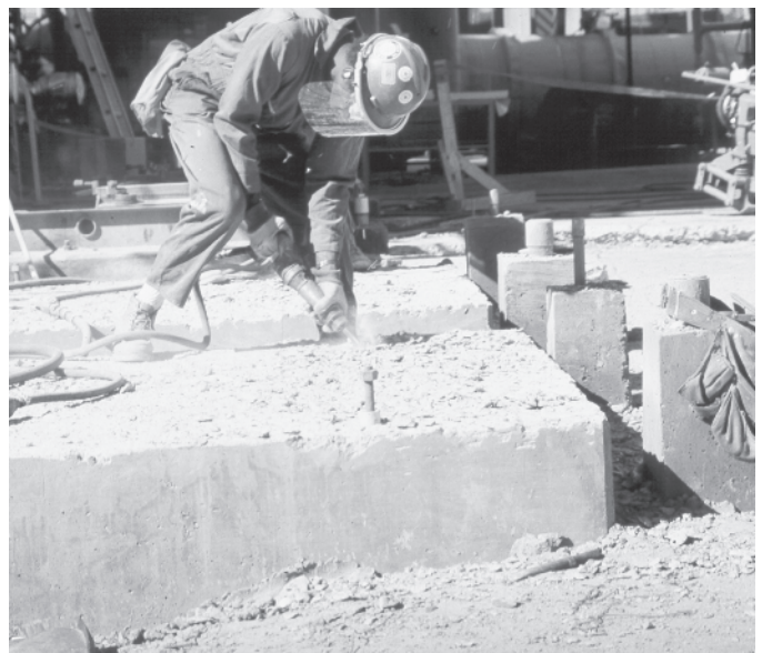
Figure 3-26: Foundation chipping in progress
