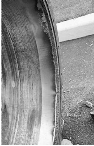
FIGURE 4 Galvanic corrosion is evident on this pump section. Note the high corrosion rate on the interior diameter of the carbon steel flange that is attached to the stainless steel shroud.
