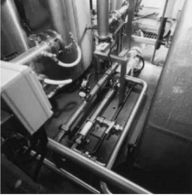
FIGURE 7A through C Typical installations of a progressive cavity hygienic pumps (Mono Pumps, Ltd.)
