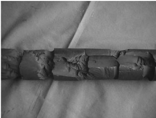
FIGURE 21 The corrosion erosion of a carbon steel shaft that was damaged in an ultra-pure water service after approximately six months
