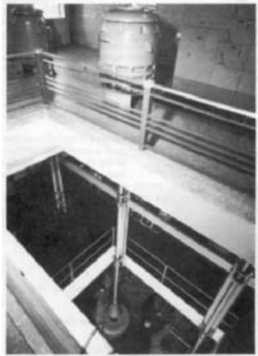
FIGURE 22 Sections of flexible shafts and intermediate guide bearings used to transmit torque from motor located above flood elevation to pump located below ground (Flowsolve Corporation)
