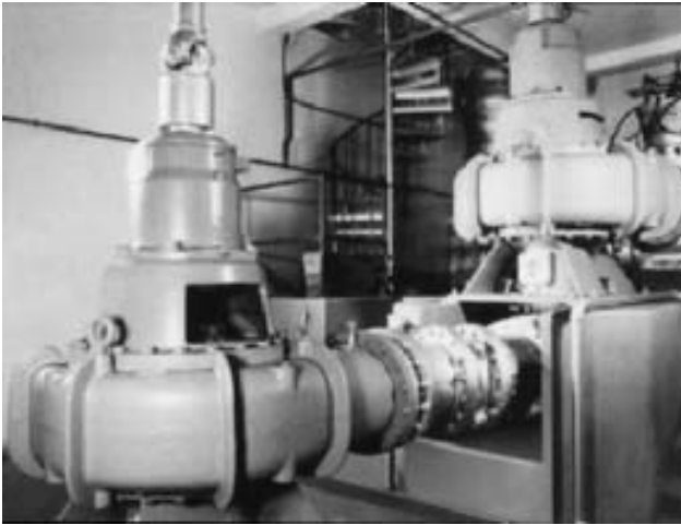
FIGURE 103 An installed vertical sewage pump similar to that shown in Figure 102 (Flowserve Corporation)
