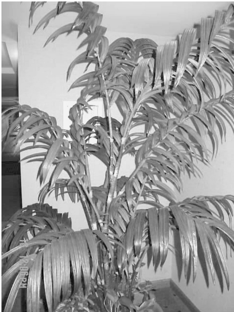
EXHIBIT 14.3 Obstructed Remote Annunciator. (Source: Hughes Associates, Inc., Warwick, RI)
