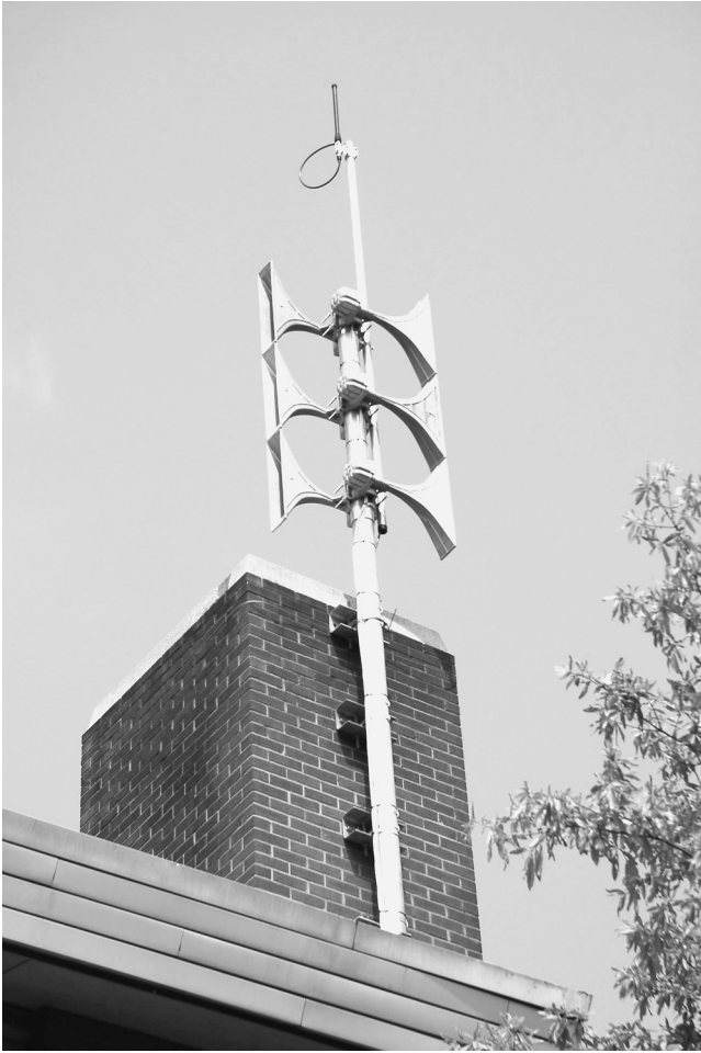
EXHIBIT 24.11 Mounted High Power Speaker Array. (Source: Cooper Notification, Long Branch, NJ)
