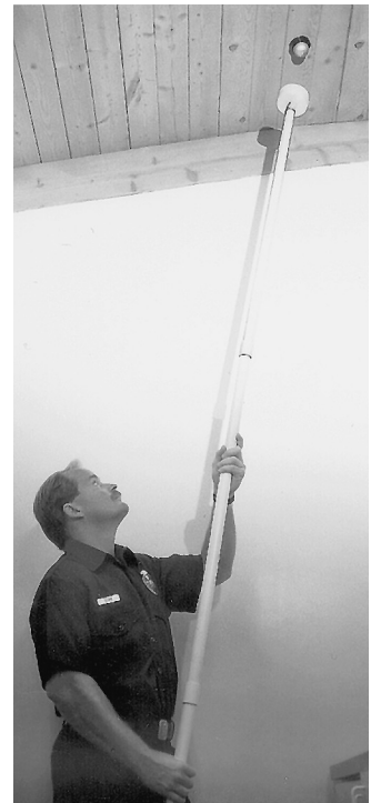
EXHIBIT 14.17 Technician Using a Heat Detector Tester. (Source: Home Safeguard Industries, Inc., Rolling Meadows, IL)
