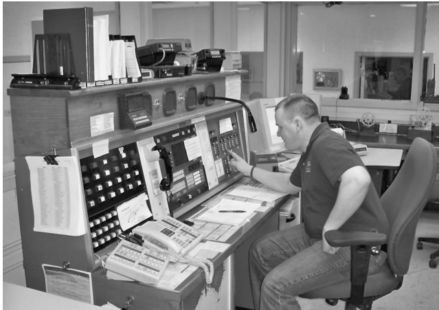
EXHIBIT 26.8 A Public Emergency Services Communications Center Equipped to Receive Signals as a Remote Station Supervising Station. (Source: James A. Spear, P.E., LeRoy, NY)
