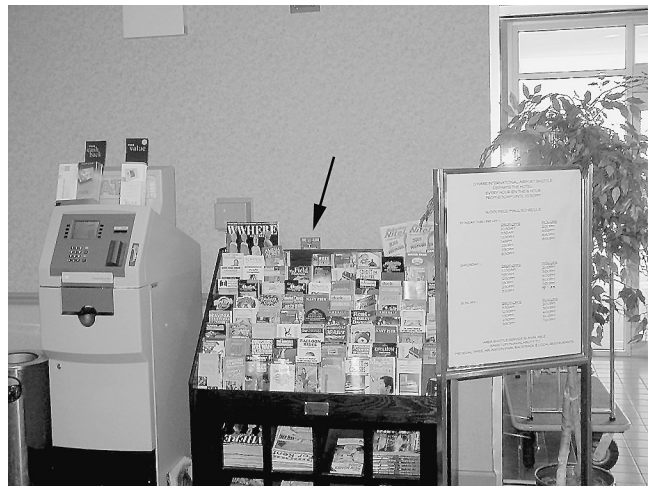
EXHIBIT 14.4 Concealed Manual Fire Alarm Box. (Source: Automatic Fire Alarm Association, Inc., Lake Mary, FL)
