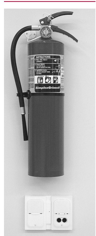
EXHIBIT 23.7 Wireless Fire Extinguisher Monitoring Device. (Source: MIJA Inc., Rockland, MA)
