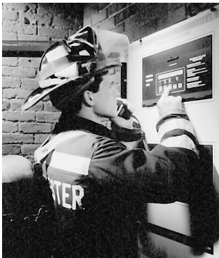
EXHIBIT 3.31 Fire Official Using Paging System. (Source: SimplexGrinnell, Westminister, MA)
