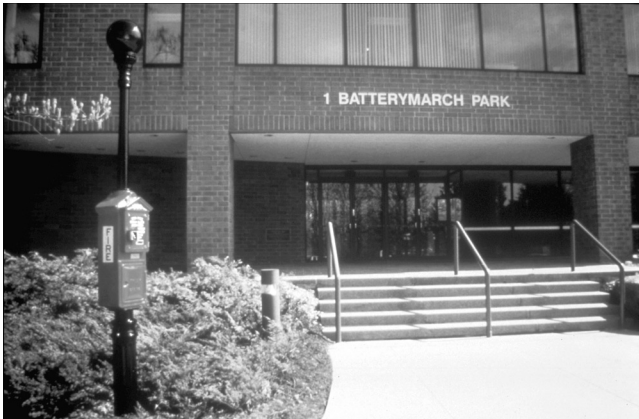
EXHIBIT 27.1 Public Emergency Alarm Reporting System Box 1896.
