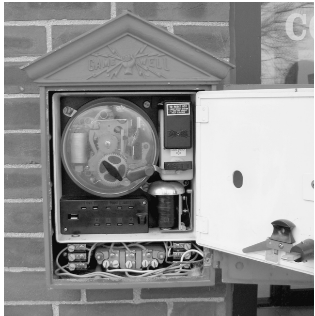
EXHIBIT 27.6 Inside View of a Master Box. (Source: Lakes Region Mutual Fire Aid, Laconia, NH; photo by Debbie Kardaseski)
