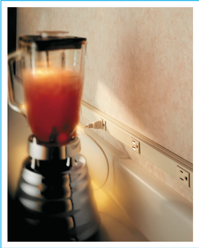
Exhibit 100.10 Multioutlet assembly installed to serve countertop appliances. (Courtesy of The Wiremold Co.)
