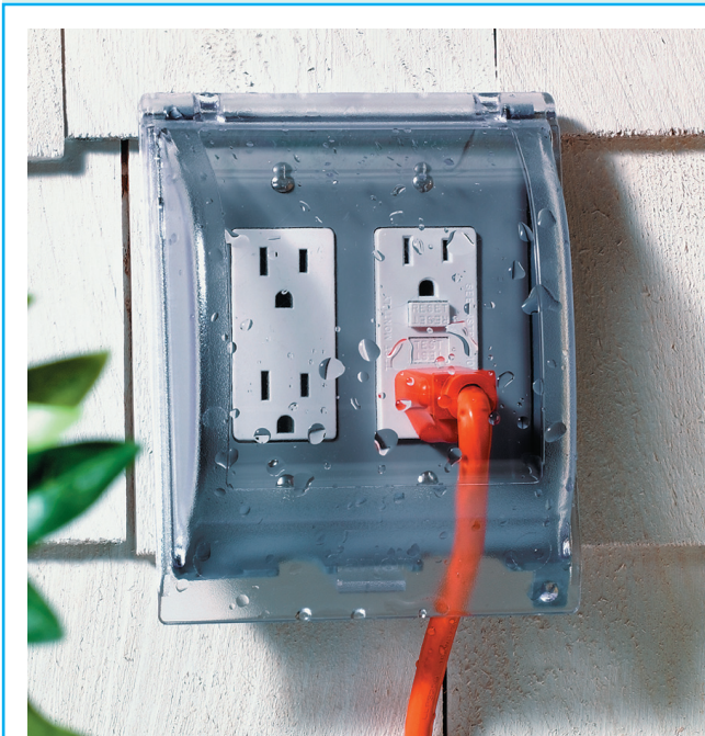
Exhibit 406.7 A two-gang weatherproof cover suitable for use in wet locations. (Courtesy of Carlon®, Lamson & Sessions)
