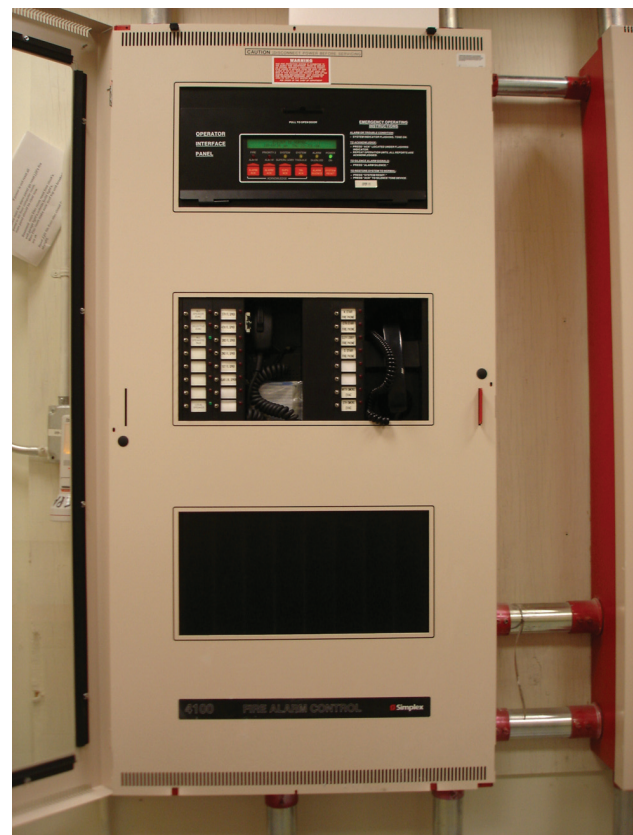
Exhibit 760.1 Typical fire alarm control unit.
