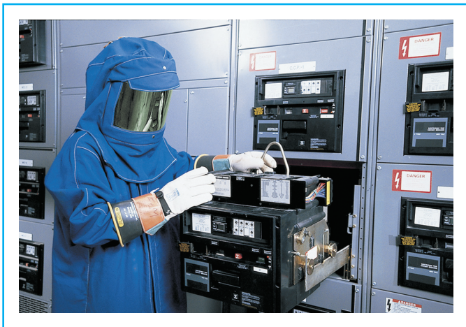
Exhibit 110.7 Electrical worker clothed in personal protective equipment (PPE) appropriate for the hazard involved.
