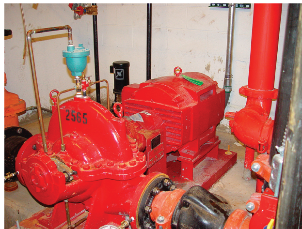
Exhibit 695.1 An electric motor specifically listed for fire pump service. (Courtesy of International Association of Electrical Inspectors)
