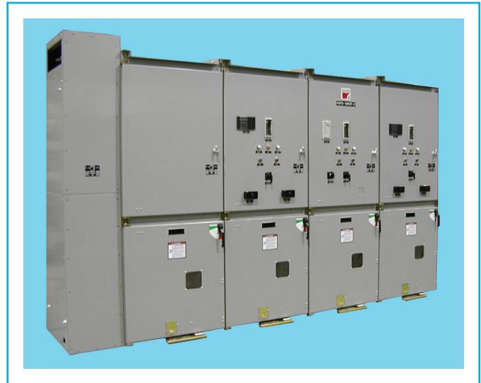
Exhibit 230.33 Metal-enclosed switchgear. (Courtesy of Square D Co.)
