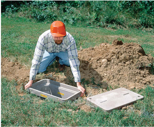
Exhibit 100.9 Example of handhole enclosure installation. (Courtesy of Strongwell)
