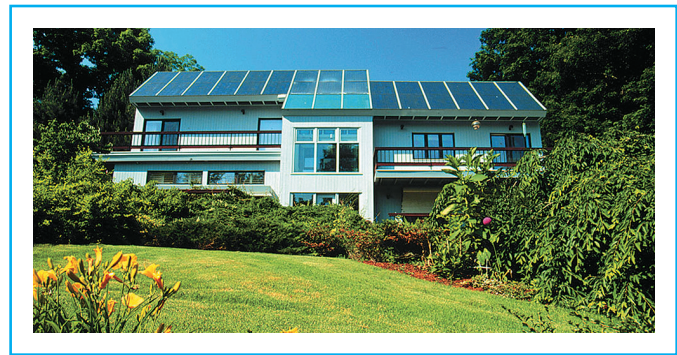
Exhibit 690.1 The south roof of a solar house. The integrated array of glass modules generates electricity directly from the sun using PV modules. (Courtesy of Solar Design Associates, Inc.)
