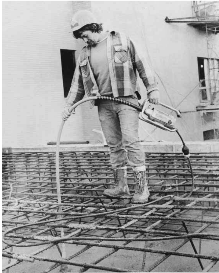
FIGURE 5.69 \frac{3}{8} in (9.5 mm) flexible shaft drives eccentric inside of steel shell to vibrate concrete; operation speed up to 13,000 rpm.
