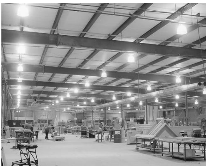
Figure 19-12. Luminaire spacing is influenced by mounting height and structural elements. It is usually desirable to coordinate luminaire location with the structural design to enhance aesthetics.
