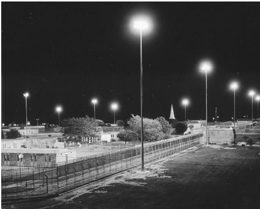
Figure 14-24. High-mast lighting for a prison yard.
