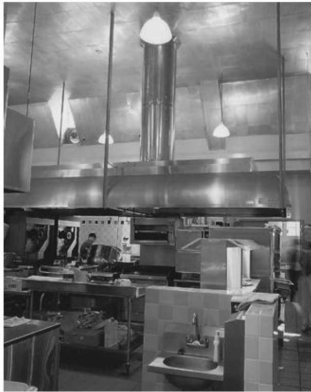
Figure 13-13. This university food service kitchen has a bright, hygienic appearance with light levels high enough to accomplish the variety of food preparation and clean-up tasks that are performed in a kitchen.
