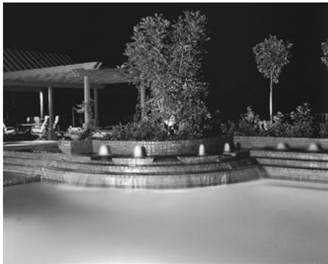
Figure 18-28. Swimming pool lighting must illuminate potential obstacles such as the edge of the pool, stairs, and landscape features such as fountains and brick terracing.
