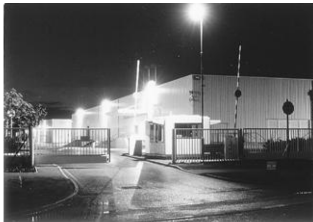
Figure 29-21. Secure entrances must be sufficiently illuminated to enable inspection of visitors or automobiles.
