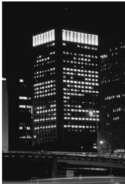
Figure 21-13. Architectural lighting can emphasize an exterior's vertical structural elements.
