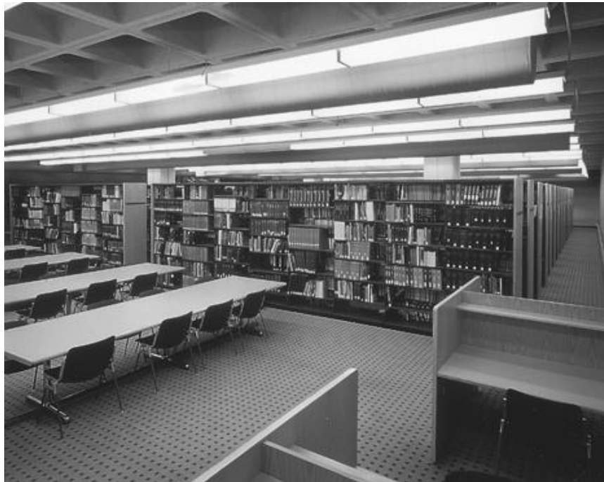
Figure 12-6. Open-access stacks are lighted with rows of fluorescent luminaires parallel to the stacks.
