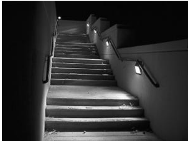
Figure 21-7. Effective hazard lighting on stairs. This lighting is unidirectional, emphasizing stair treads.
