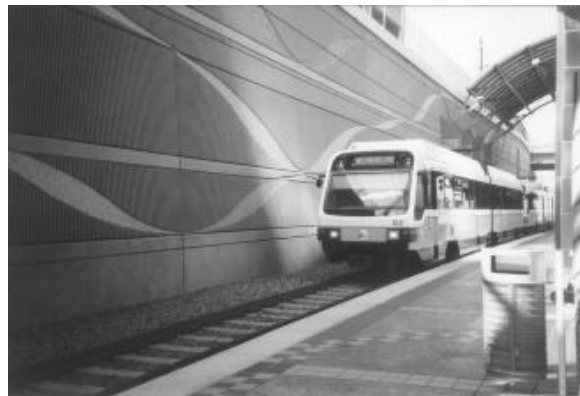
Figure 23-15. Rail stations can be well lighted for after-dark operation so that the lights do not trespass onto neighboring property. Note that the overhead lighting is directed toward the station. Adequate lighting and aesthetic elements such as the distinctive wall design contribute to passenger comfort, safety, and appeal.
