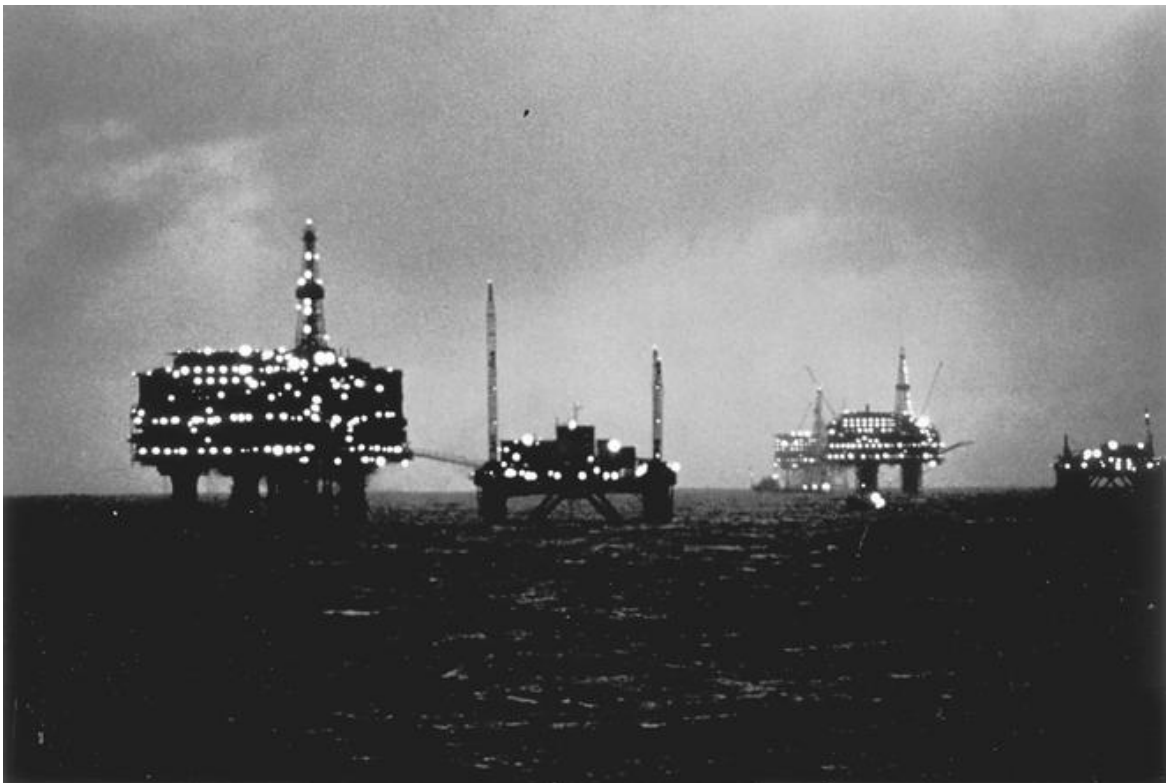
Figure 23-31. Nighttime illuminance permits offshore oil rigs, such as these North Sea production platforms, to operate around the clock. Care must be taken to avoid masking obstruction and navigation lights.
