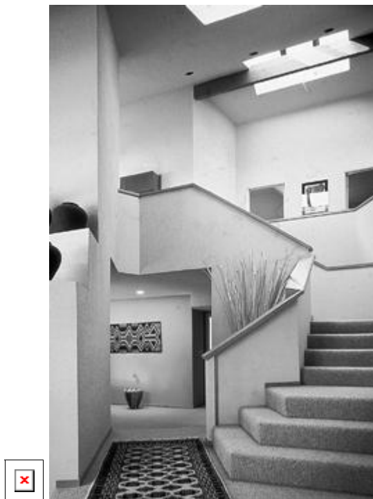
Figure 18-5. Left, a three-dimensional effect was created for the lighting of this hallway. Three recessed PAR-30 spotlights were used to wash the wall of the upper hallway and give depth to the view. The open passageway was lit with wall-mounted up/down fluorescent lamp luminaires. A low voltage incandescent strip was used to light the railing. The bottom step of the staircase was illuminated with a downlight, while the dried reeds were illuminated with uplight. This lighting scheme plays with various brightnesses and emphasizes three-dimensional planes and depths. Right, a daytime view of the same hallway. While the skylight is pronounced, the three-dimensional features of the lighting scheme are not as noticeable.
