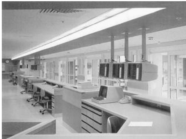
Figure 16-2. Lighting at a nurses' station is multilevel, to allow for a higher illumination during the day and a lower level at night. The lighting is designed for the critical task of reading patient information from the computer screen. Undercounter task lights also function as night lights.
