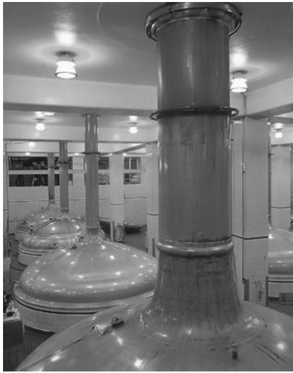
Figure 19-10. Wide distribution HID luminaires can be effective at low mounting heights if glare is controlled by good luminaire design and light background colors.
