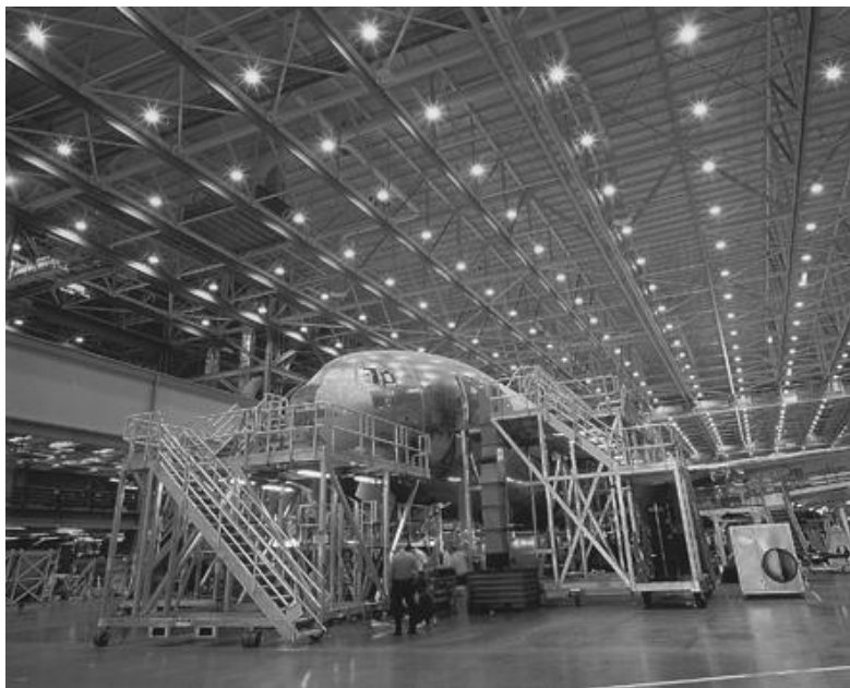
Figure 19-27. Widespread high-bay HID luminaires with uplight provide proper horizontal and vertical illuminance for large parts assembly while lighting the ceiling and walls to improve environmental surroundings.
