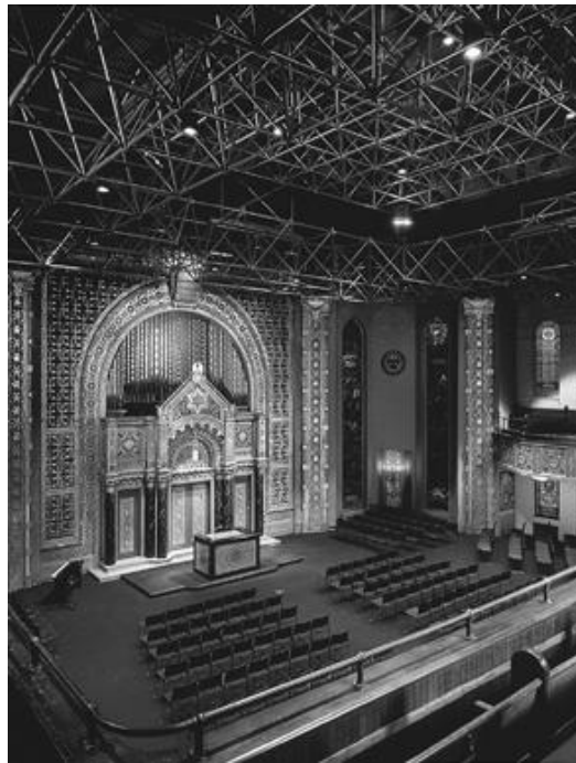
Figure 14-19. Synagogue lighting. Accent lighting highlights the holy ark and bema. Downlights mounted on a triangulated space frame illuminate the congregational area.
