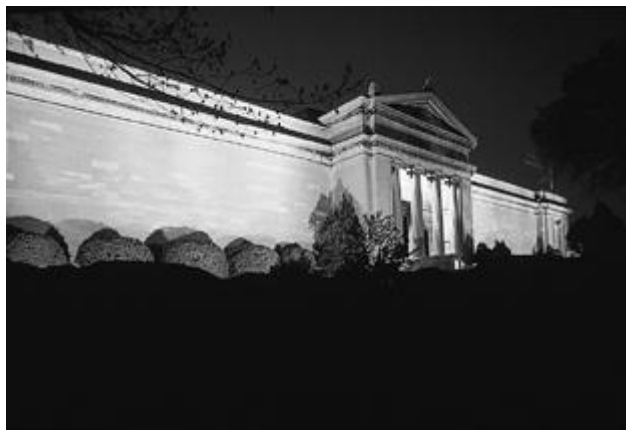
Figure 21-20. Good vertical surface illuminance without hot spots
