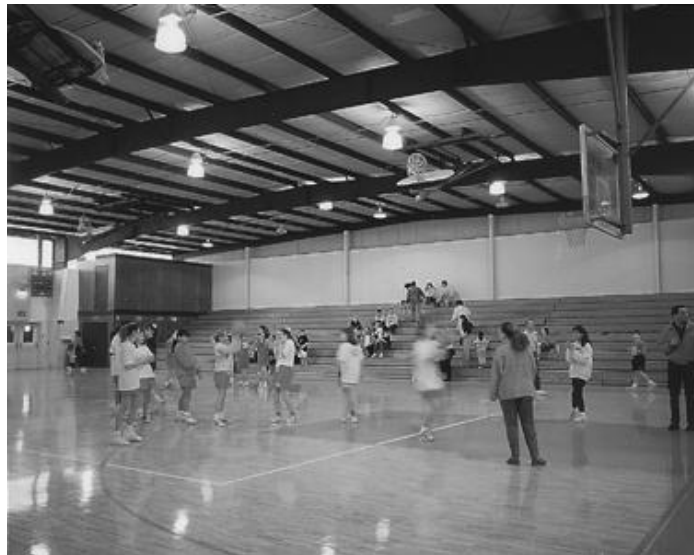
Figure 12-8. A gymnasium lighted with surface-mounted HID luminaires.
