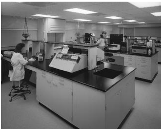
Figure 16-11. High color rendering fluorescent lighting is used in this hospital tissue laboratory.
