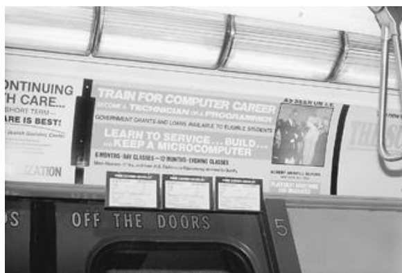
Figure 23-12. Continuous rows of linear fluorescent luminaires with prismatic diffusers light the car and opaque advertising cards over the car windows.
