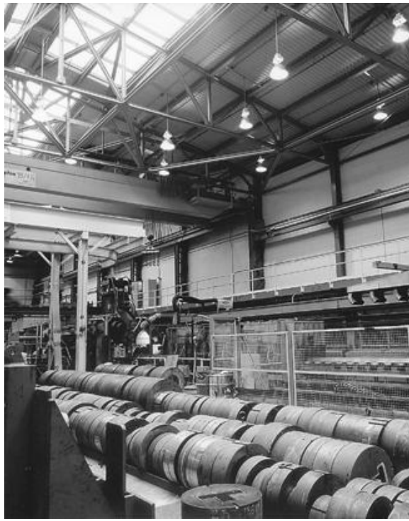
Figure 19-5. Uniform lighting in a location such as this allows flexibility in the use of the space without the expense of relocating luminaires.
