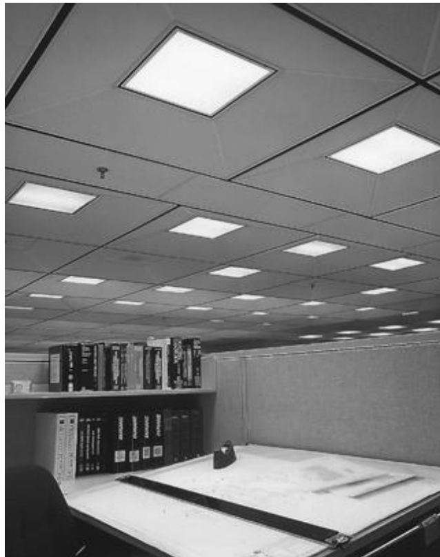
Figure 11-10. Direct lighting from a fluorescent system that provides good general illumination as well as adequate light for working at the drafting table.
