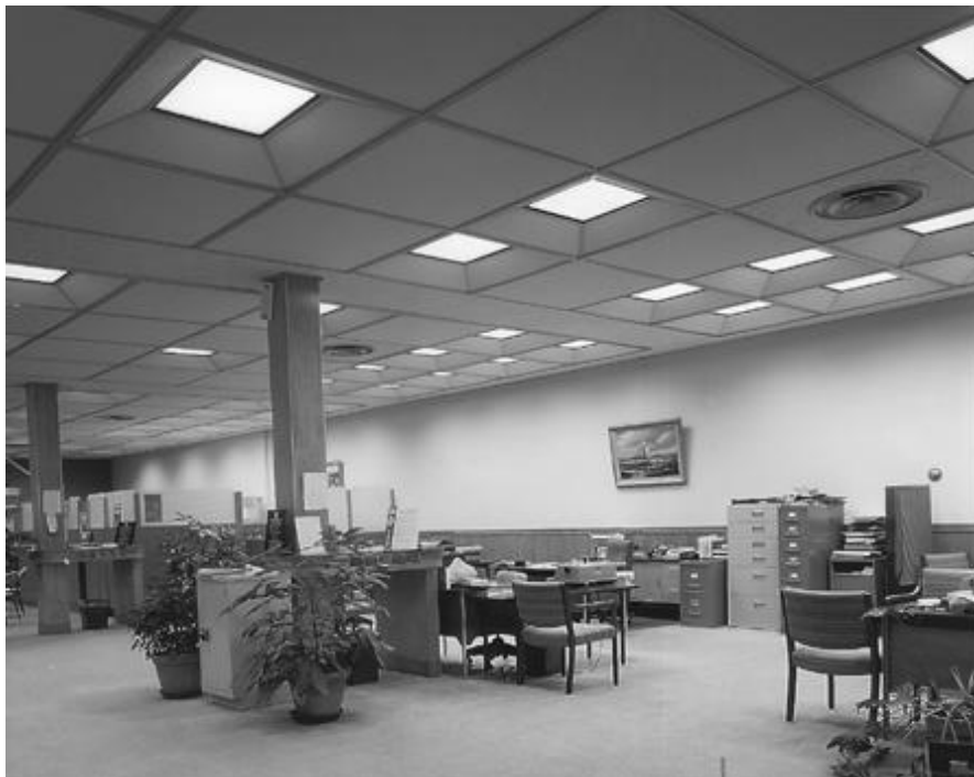
Figure 11-21. A modern banking facility with general illumination provided by fluorescent lighting.
