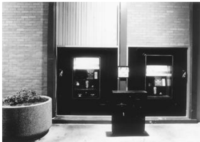
Figure 11-22. ATM illuminated with a side-mounted HID light source that provides proper lighting to the user of the machine with no veiling glare. In addition, the light source is properly directed to highlight such potential obstructions as the desk and the planter.
