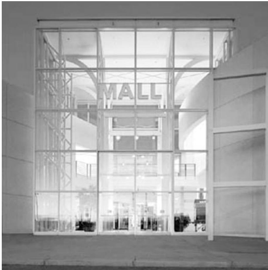
Figure 17-24. High-reflectance surfaces and special lighting of walls and ceilings help shoppers find main mall entries.
