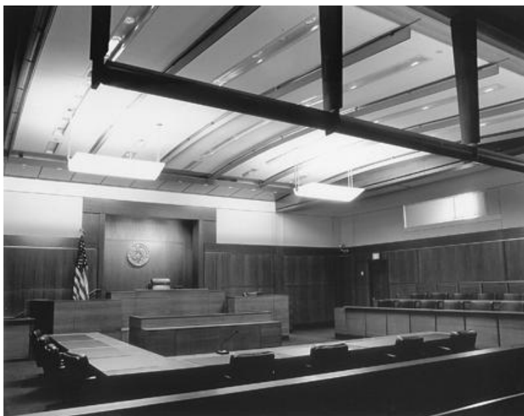
Figure 14-23. The 15 courtrooms in the Mark O. Hatfield U.S. Courthouse are lighted with a combination of 32-watt T-8 fluorescent lamps with electronic ballasts plus 50-, 60- and 100-watt halogen lamps. The lighting is controlled by a system on the judge's bench.
