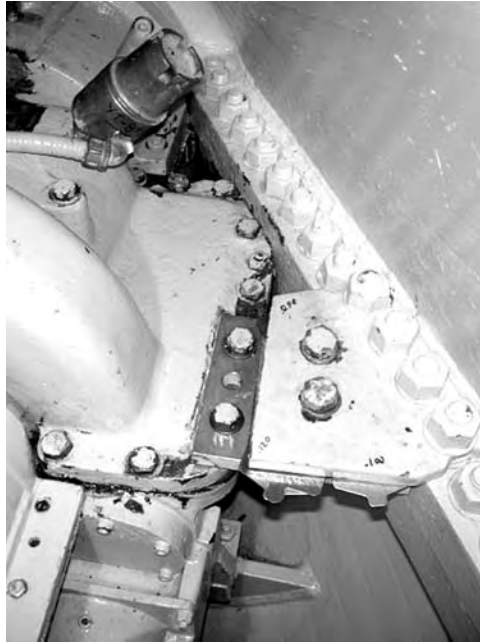
FIGURE 5.54 Soft foot shims installed on turbine bearing lateral support plates.
