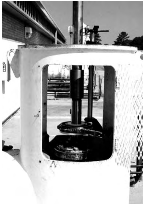
FIGURE 21.38 Measure the eccentricity at the lower end of the pump shaft.
