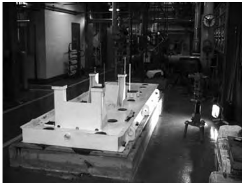
FIGURE 3.60 Jig transit set up to observe final elevations on foot pads.
