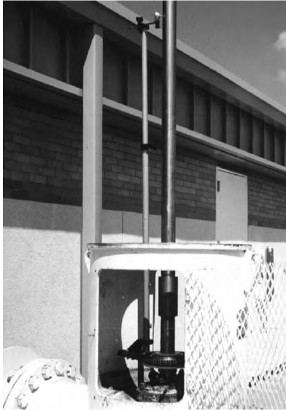
FIGURE 21.39 Measure the eccentricity at the upper end of the pump shaft.
