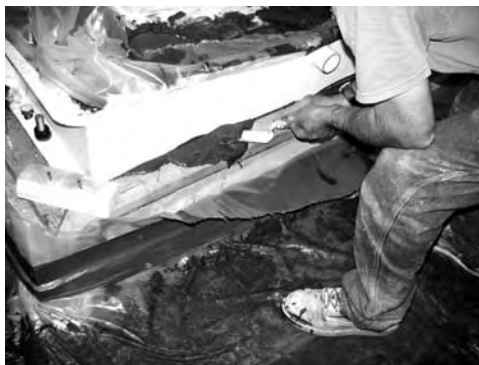
FIGURE 3.55 Scraping off the excess grout while still in the putty stage.
