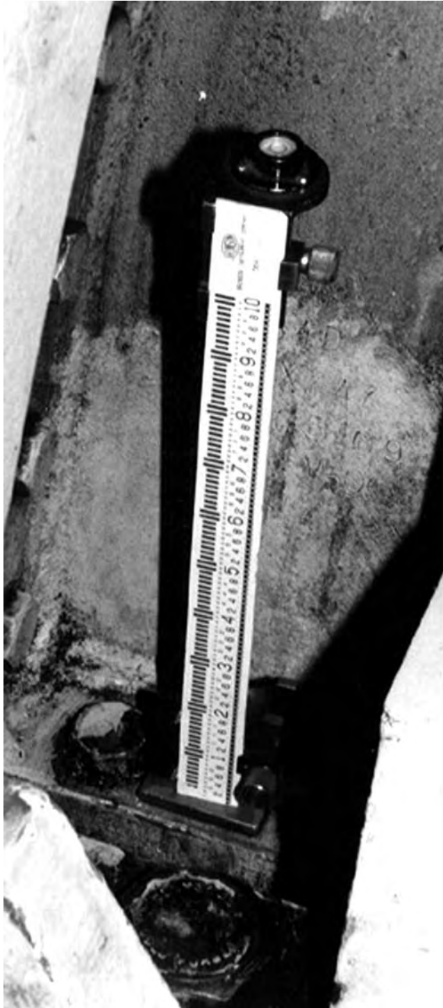
FIGURE 6.13 Scale targets mounted on an electric generator bearing.
