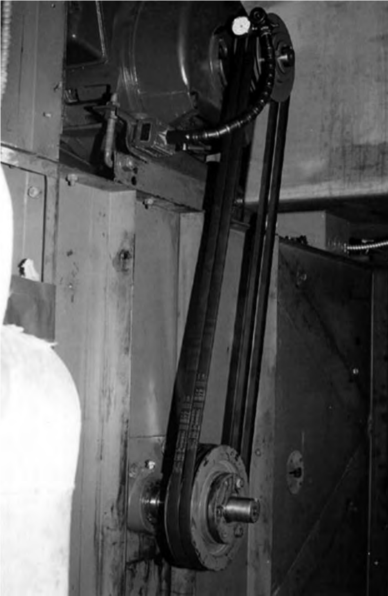
FIGURE 18.14 Rim runout check on sheave.
