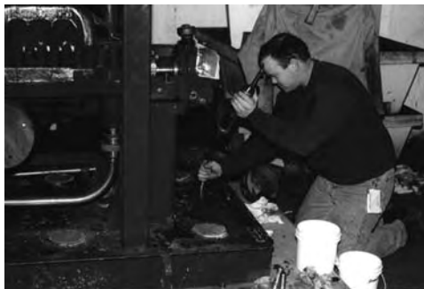
FIGURE 3.24 Injecting epoxy-based grout into voids in baseplate.
