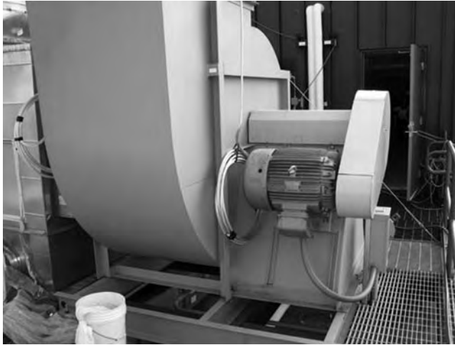
FIGURE 21.46 Belt-driven fan.
