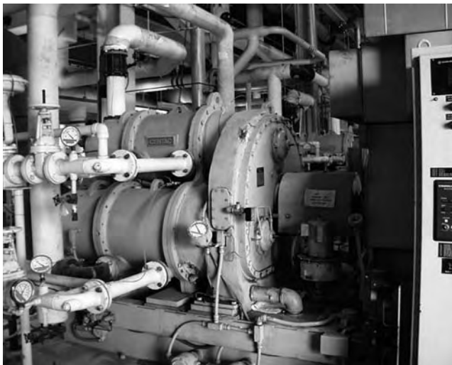
FIGURE 21.53 Multistage bullgear-driven compressor.
