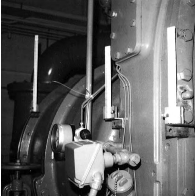
FIGURE 6.14 Scale targets mounted on compressor casing near their centerline of rotation.
