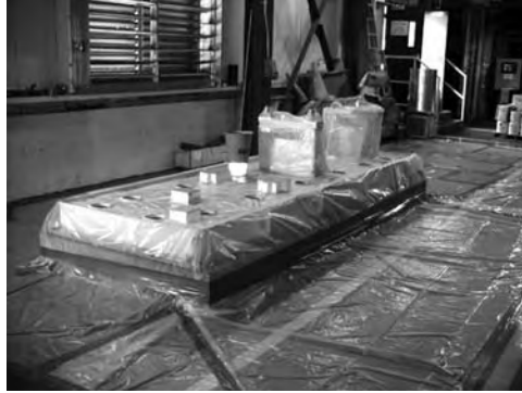
FIGURE 3.46 Protecting the baseplate and surrounding area with plastic covering.
