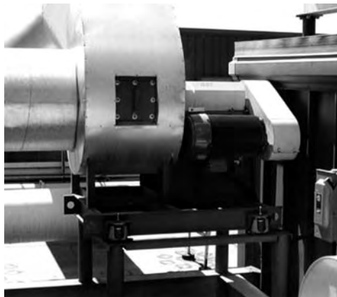
FIGURE 3.3 Frame supporting a belt drive fan.
