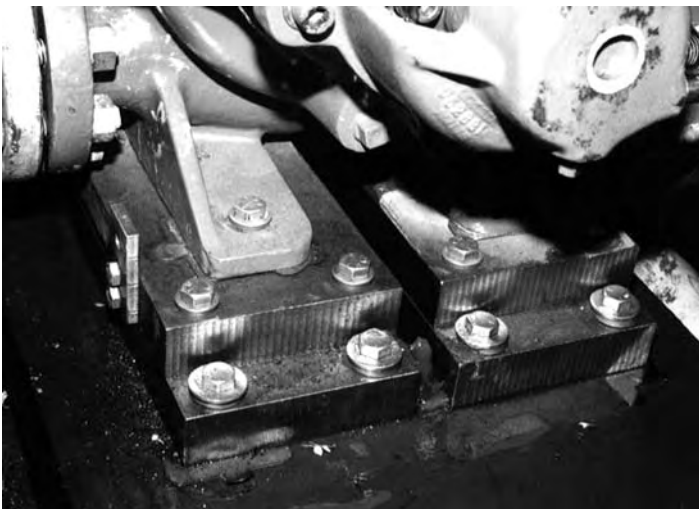
FIGURE 3.6 Weak structural steel was replaced with solid plate on this baseplate.
