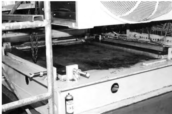
FIGURE 5.44 Sole plates cleaning under motor shown in Figure 5.42.
