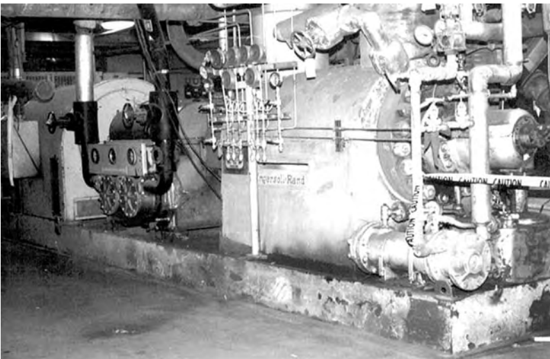
FIGURE 17.2 Motor-fluid drive-pump drive system.
