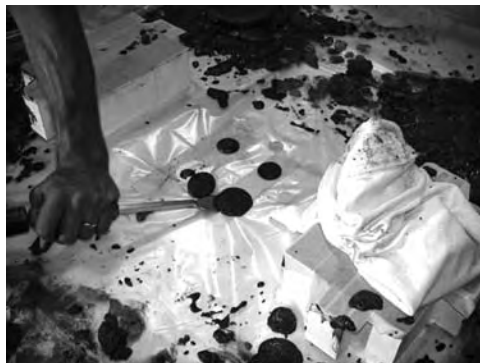
FIGURE 3.57 Chiseling off the excess grout.
