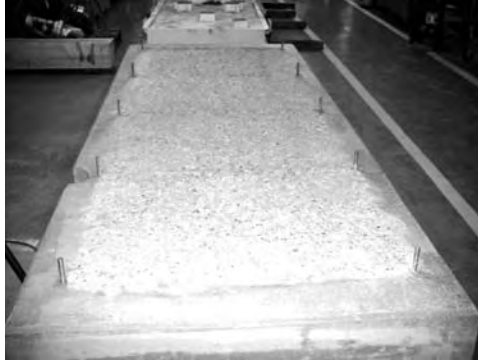
FIGURE 3.26 Scarifying the top surface of a concrete foundation.
