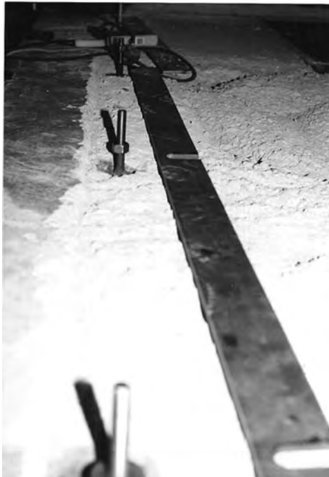
FIGURE 3.7 Soleplate being prepared for grouting.
