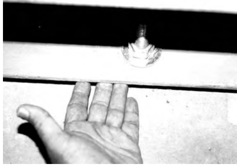
FIGURE 3.66 Fan frame mistakenly designed with no soleplates imbedded in concrete resulting in no contact between underside of frame and top of concrete in the inertia block.
