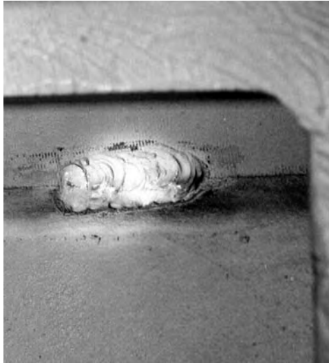
FIGURE 5.19 Cracked weld on machine housing.
