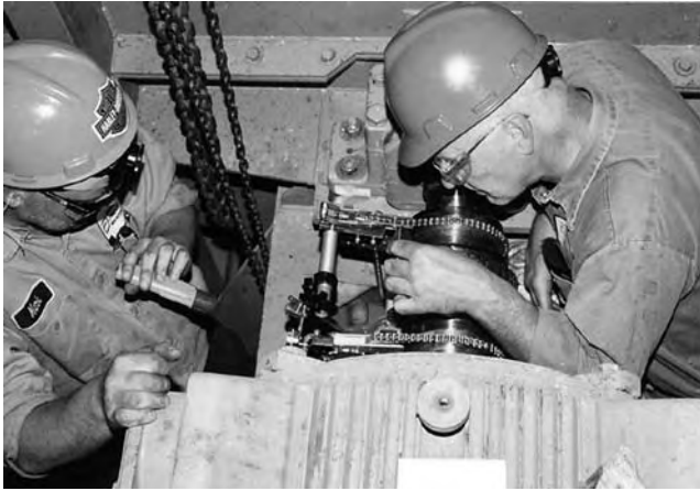
FIGURE 21.48 Aligning a direct-driven fan.
