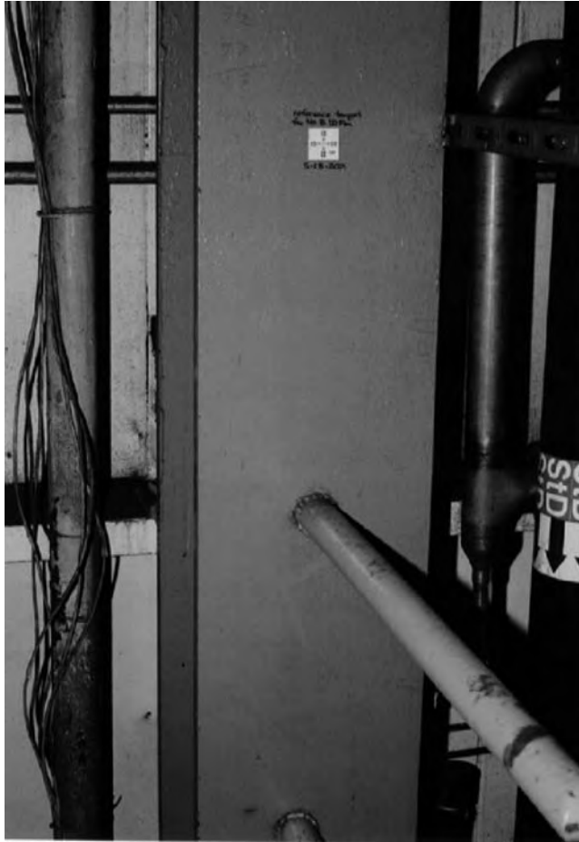
FIGURE 16.51 Adhesive-backed target attached to I-beam.
