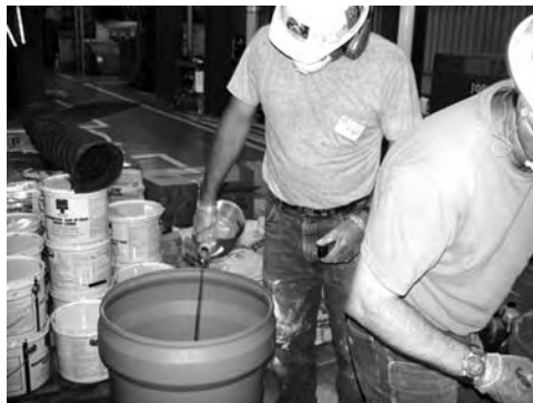
FIGURE 3.47 Mixing the grout contents.
