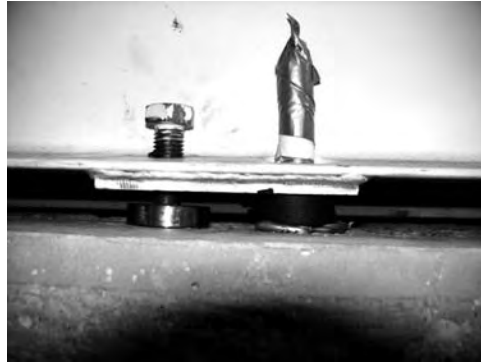
FIGURE 3.39 Close-up of jackscrew and anchor bolt.
