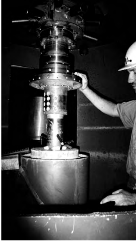
FIGURE 21.21 Centering the pump shaft in its upper bushing.
