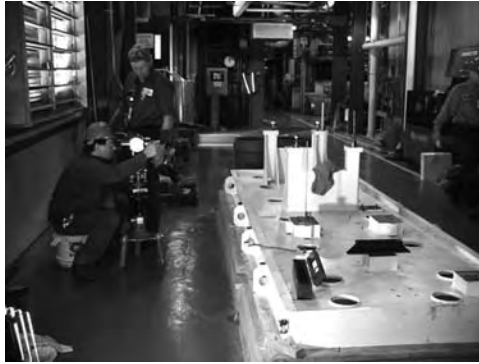
FIGURE 3.42 Double checking elevations with two independent observers.
