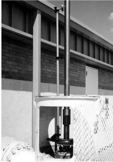
FIGURE 5.28 Measuring runout on the same drive shaft near the top of the shaft.
