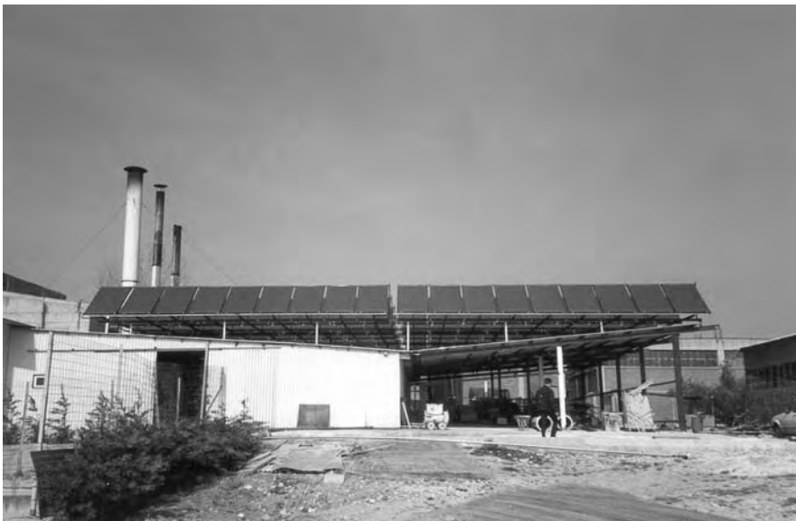
FIGURE 20.38 Alpino SA, dairy industry, Greece. Installed capacity: 518 kW th . (From Alpino SA, Greece. With permission.)
