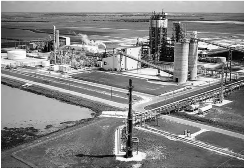
FIGURE 6.13 The 250-MW coal gasification plant at the polk plant of Tampa Electric.
