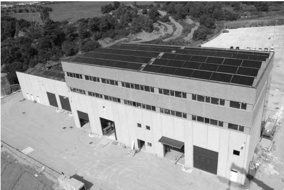
FIGURE 20.40 Parking service Castellbisbal SA, container washing, Spain. Installed capacity: 357 kW th . (From Aiguasol Engineering, Spain. With permission.)
