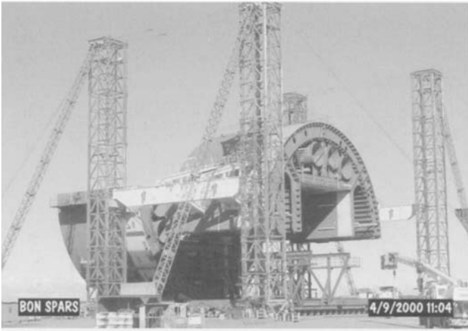
Figure 7.79 Lifting of upper half-section (Technip Offshore)
