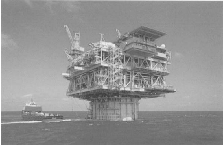
Figure 7.10 Three level topsides deck (Diana DDCV, Courtesy of EXXONMOBIL)
