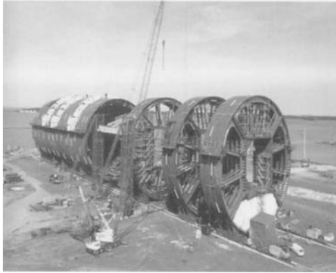
Figure 7.81 Construction of the spar (Technip Offshore)
