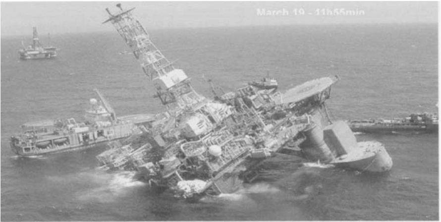
Figure 1.7 Accident of P-36 converted semi-submersible after flooding in one column [Barusco, 2002]
