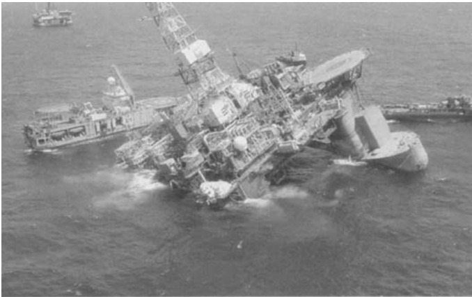
Figure 7.19 P-36 converted semi-submersible after flooding in one column (Barusco, 2002)
