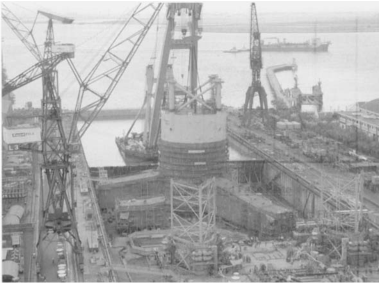
Figure 7.134 Seastar® Matterhorn platform in dry dock (SBM Atlantia)
