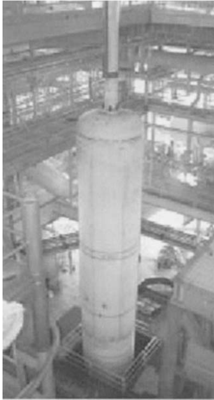
Figure 7.67 Buoyancy can being installed (Technip Offshore)
