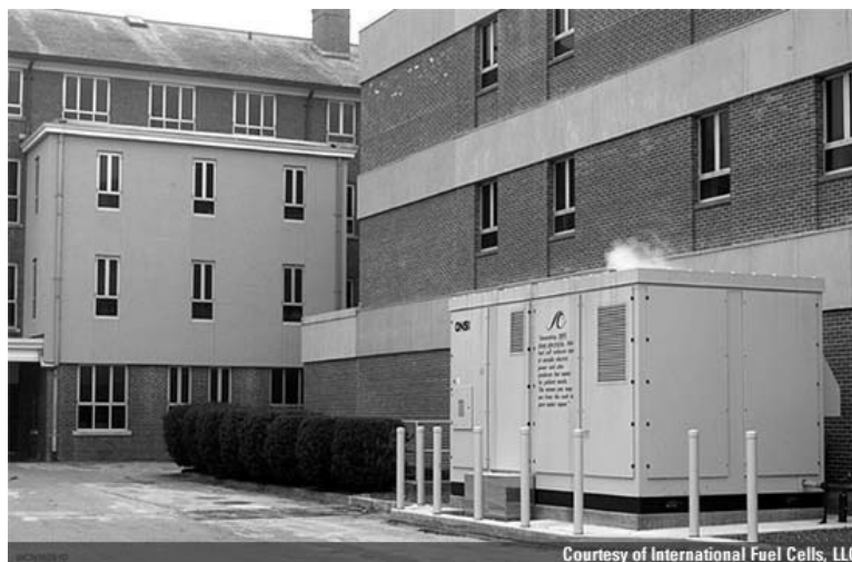
Fig. 20.10 Photograph of PC25 fuel cell unit at South County Hospital, Wakefield, RI, USA. (Courtesy of International Fuel Cells Inc.)
