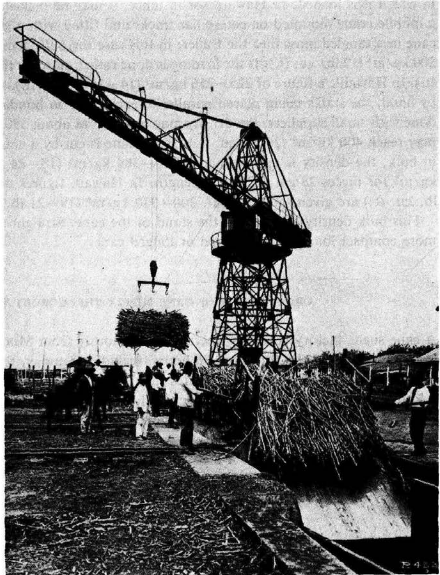
Fig. 1.2. Lifting a bundle of cane
