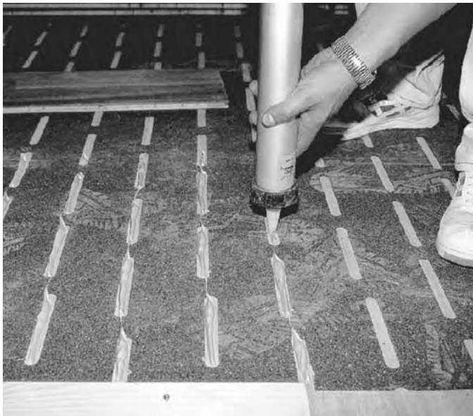
Figure 104: Application of adhesive in noise-dampening floor bonding.
