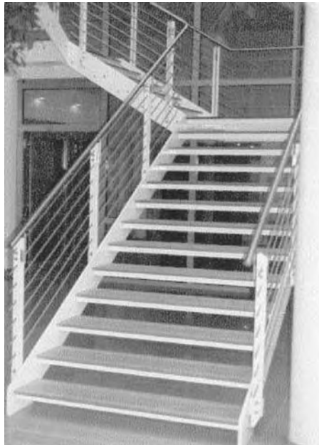
Figure 112: Elastically bonded stairs.
