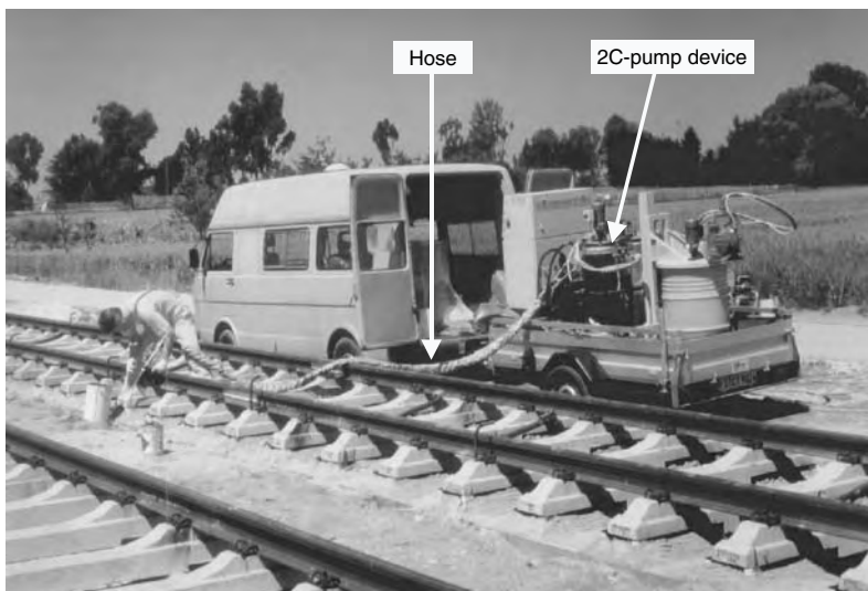
Figure 116: Application with 2C-pump device at construction place.
