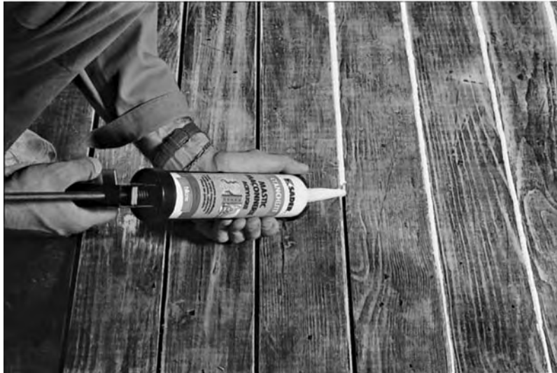
Figure 14: Cartridge and gun application of an adhesive/sealant.
