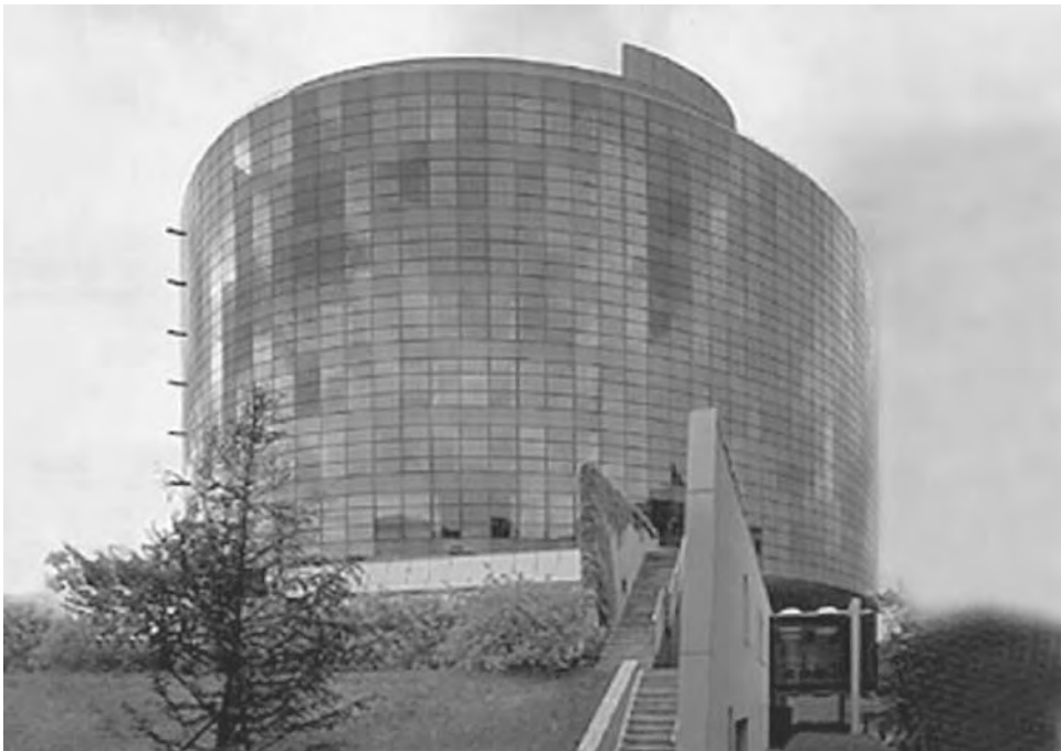
Figure 2: Example of structural glazing of facades, Berlin. This requires a flexible bond and seal.
