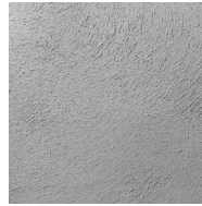
Sand-aggregated float finish
