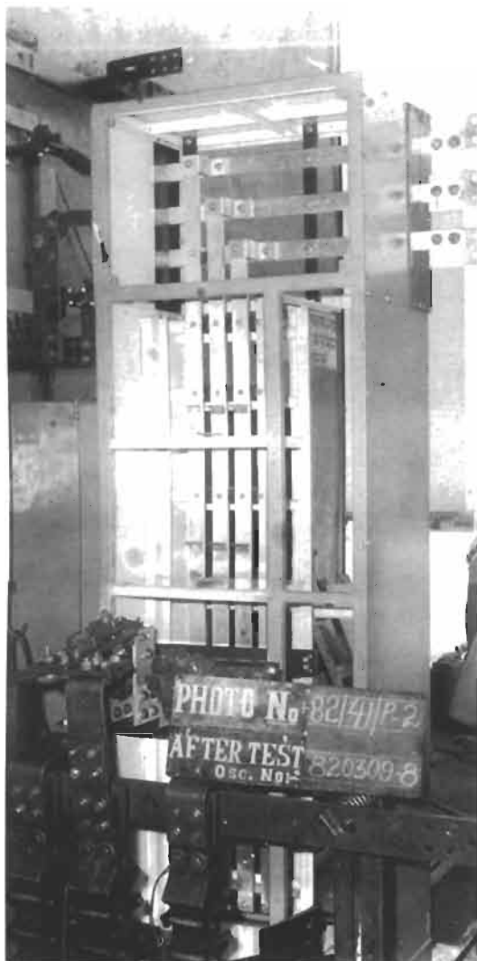
Figure 14.8 A motor control centre (MCC) after short-circuit test at CPRI
