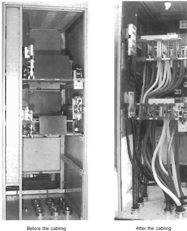
Figure 13.33 Arrangement of gland plates
