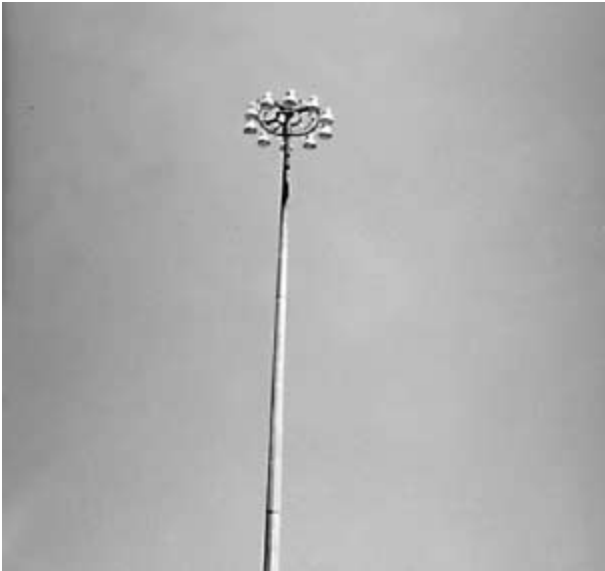
High-mast lighting can provide even illuminance levels.
