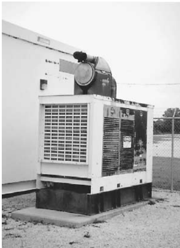
Diesel engine generator set.
