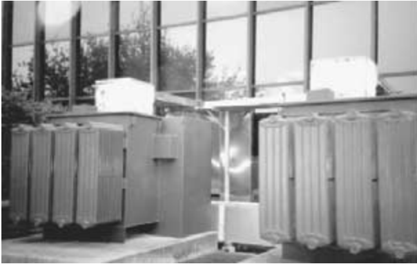
Liquid-filled transformers can carry extra power when fitted with cooling stages.
