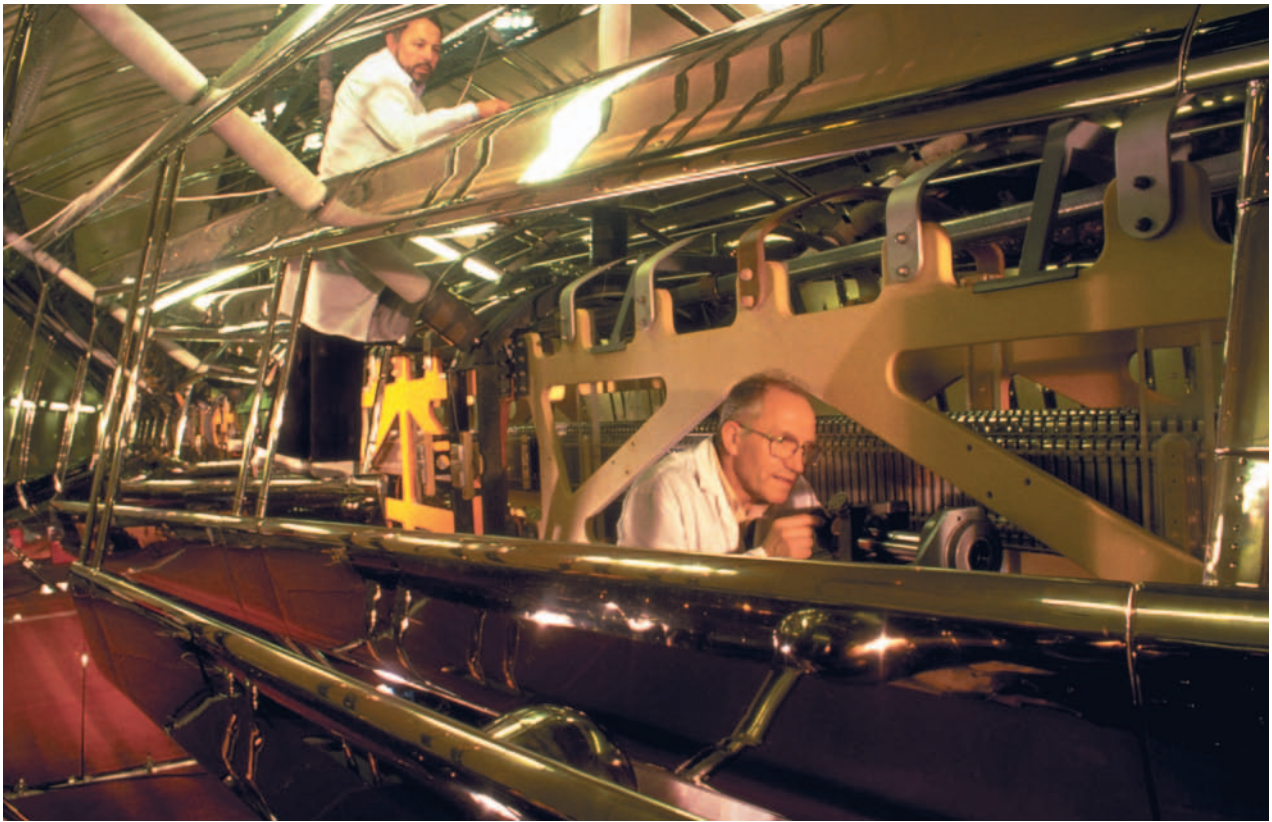
The Vivitron electrostatic particle accelerator under construction at the Centre des Recherches Nucleaires, Strasbourg, France. Vivitron, the largest Van de Graaff generator in the world, can generate a potential of up to 35 million volts. The accelerator will be used to fire ions of elements such as carbon at other nuclei. Under the right conditions this creates superdeformation, a relatively stable state in which the rotating nuclei have an elliptical form. Gamma rays given off by these nuclei reveal much about the internal structure of the nucleus. Photograph by Philippe Plailly/Eurelios. National Audubon Society Collection/Photo Researchers, Inc. Reproduced by permission.
