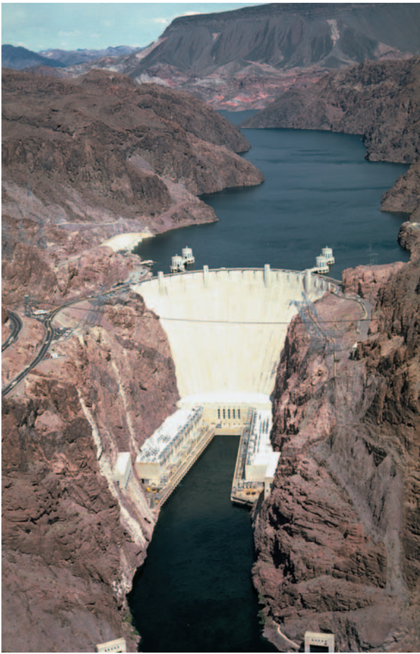
Hoover dam from downstream looking toward the east at the face of the dam. The Colorado River is in the foreground. The dam is 725 ft (221 m) high and impounds enough water in Lake Mead to cover the state of New York up to 1 ft (0.3 m) deep. Photograph by Roy Morsch. Stock Market. Reproduced by permission.
