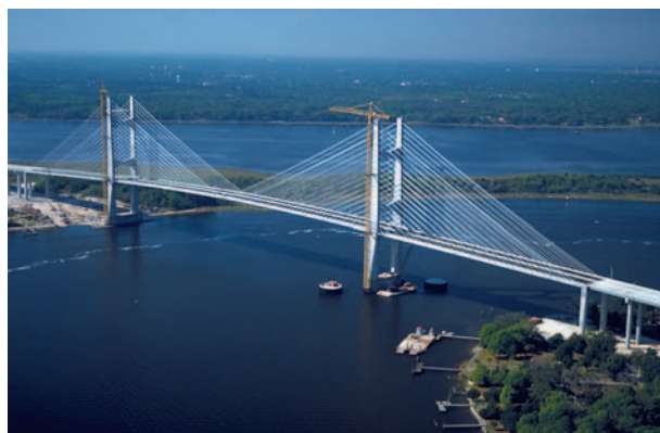
Dame Point bridge in Jacksonville, Florida, is a cable-stayed bridge. The deck is supported by cables which transmit the load to the towers. © Tom Carroll/Phototake NYC. Reproduced with permission.
