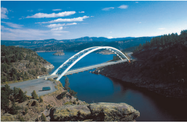
A bowstring arch bridge in Arizona. The deck is supported from the arch by hangers. The load is transmitted to the abutments by the outward thrust of the arch. JLM Visuals. Reproduced by permission.
