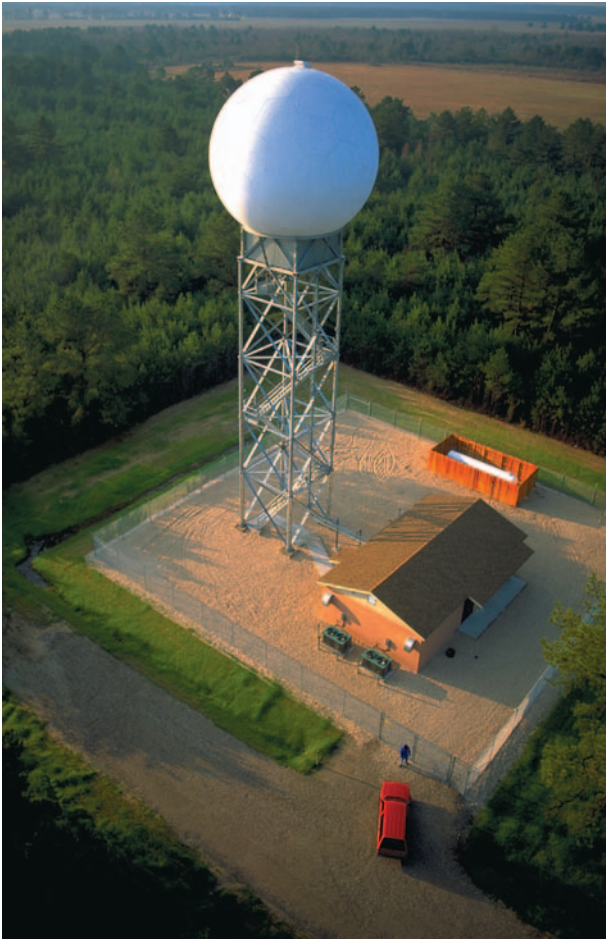
Antenna for a Doppler weather radar site. Doppler radar can be used to detect wind shear and microburst weather conditions. Photograph by Brownie Harris. Stock Market. Reproduced by permission.
