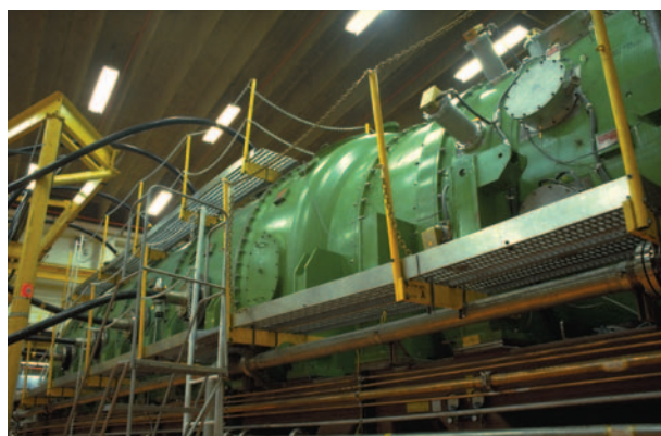
The power amplifier for the Antares fusion laser. Photograph by Ray Nelson. Phototake NYC. Reproduced by permission.
