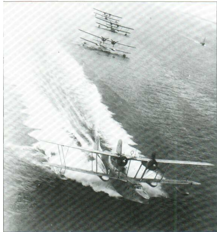
Right: A quartet of Stranraers of No. 209 Sqn at Felixstowe, Suffolk, in May 1939. Note the absence of camouflage (applied on the outbreak of war) and the underwing fuel tanks. Just before the war the squadron moved north to Invergordon.
