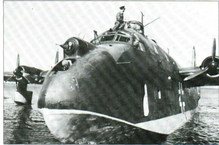
The fifth Blohm und Voss Bv 222A-O was delivered to Lufttransportstaffel (See) 222 at Petsamo, Finland, in 1943 for transport duties over the northern sector of the Eastern Front. Note the over-wing gun turret.
