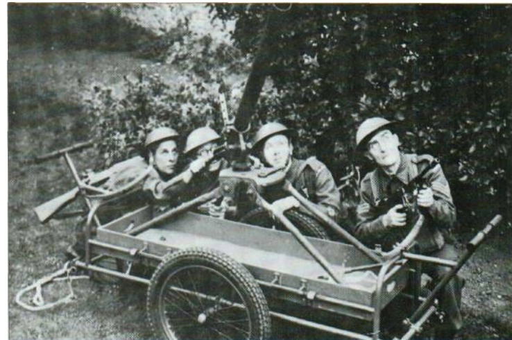
An enterprising Home Guard unit from Sussex mounted their Northover Projector on this small hand cart, and are seen optimistically using it as an anti-aircraft weapon, a role for which it was entirely unsuited. The range was far too short and the muzzle velocity of the glass grenade much too slow.
