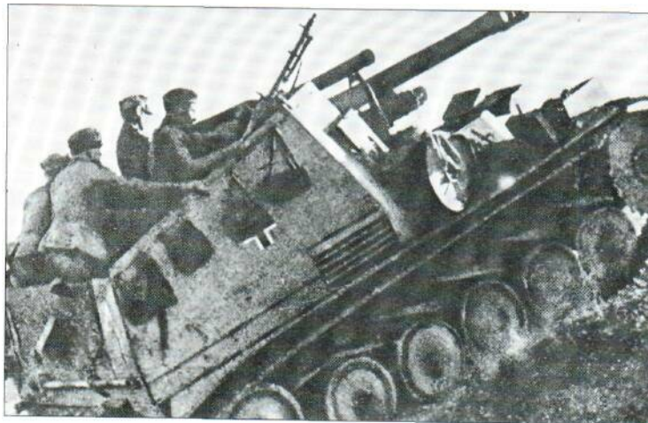
This shot of a Wespe on the move shows that the top of the fighting compartment was open but protection was provided at therear.
