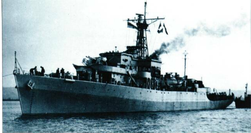
The 'Bay' class frigates were versions of the 'Loch' class optimized for Pacific operations, where escorts were more likely to be attacked from the rear. The heavy Squid system was landed in favour of the lighter but less effective Hedgehog, and AA armament was improved.
