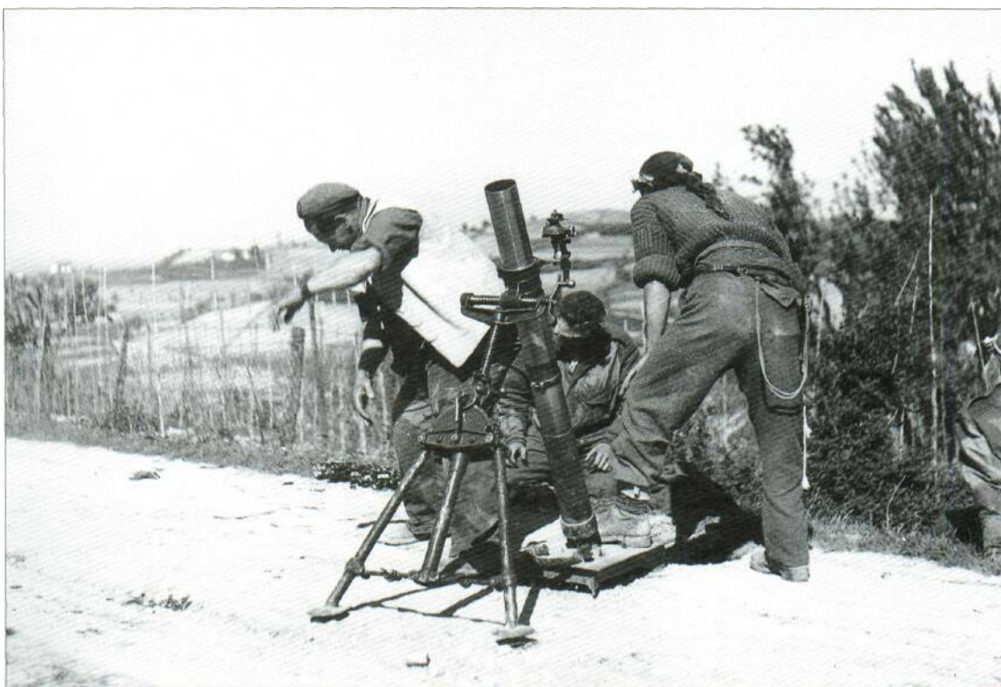
These British SAS parachutists are firing their 3in (76.2mm) ML mortar in support of a partisan attack on German forces. The mortar remains an important and powerful infantry weapon today.
