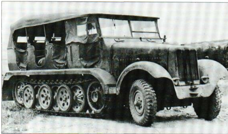
The Czech-built Praga SdKfz 6s featured longer track bogies than the Bussing-NAG models, and had different wings. They were powered
